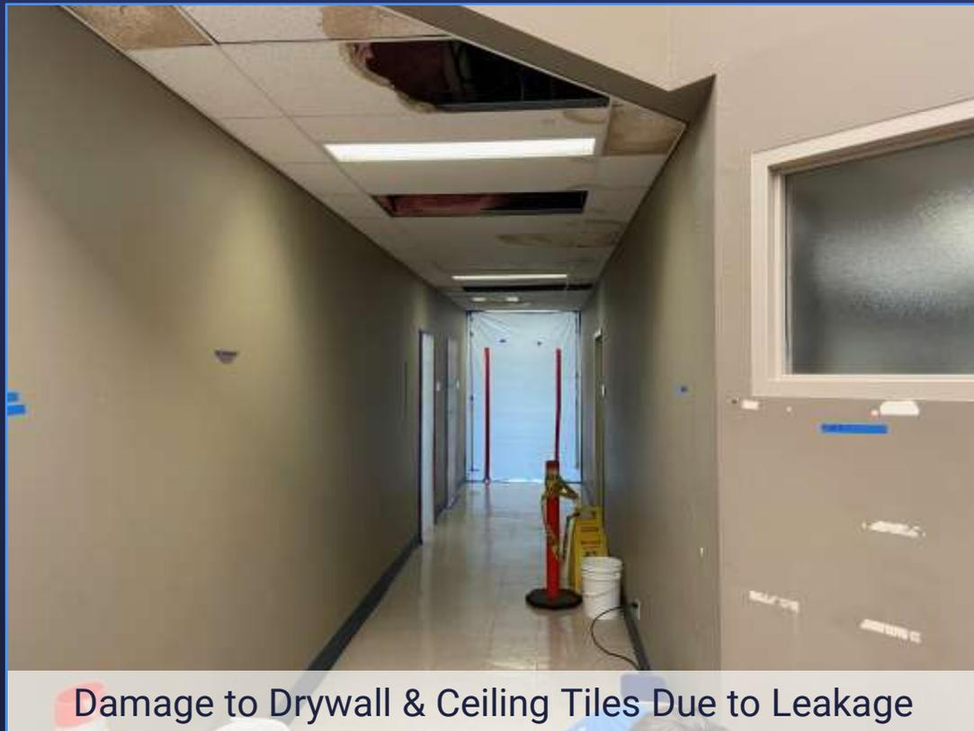
Damage to Drywall & Ceiling Tiles Due to Leakage
