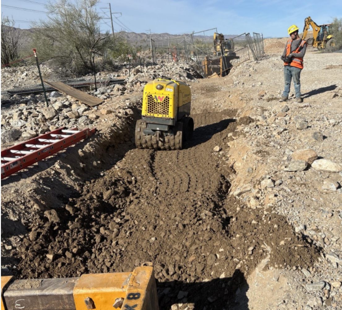
CRA Eagle and Hinds Utilities Hinds Crew using a Walk-behind Roller Compactor to Consolidate Material
