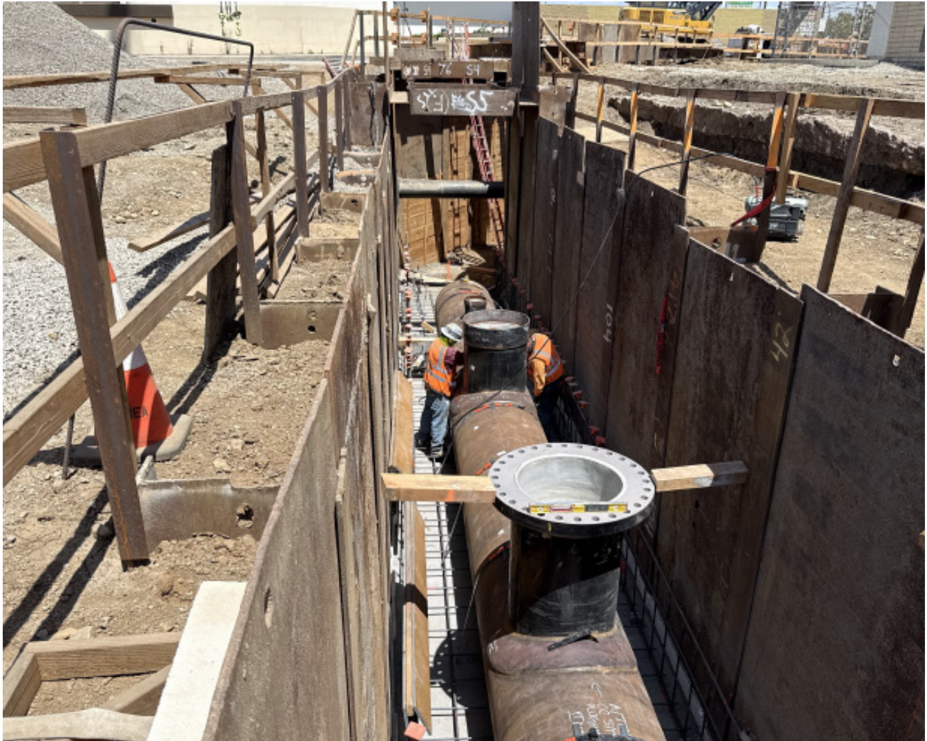
Sepulveda Feeder Pump Stations Contractor, J.F. Shea Placing the Suction Pipeline
