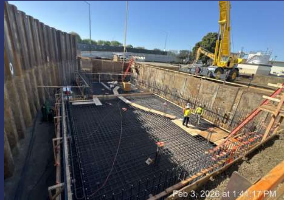
Sepulveda Pump Stations Venice PCS Site
