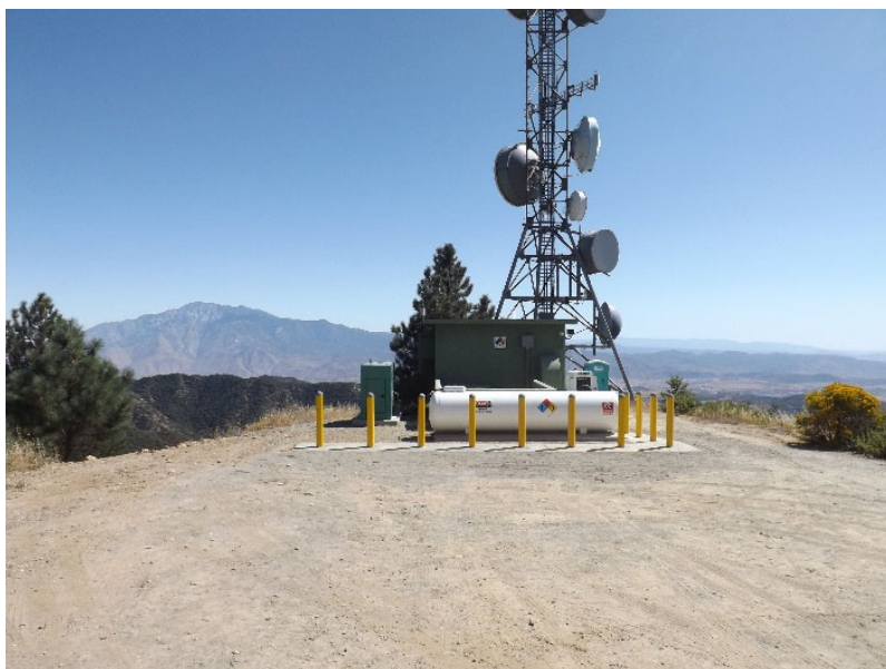
Detention Peak Communication Site
