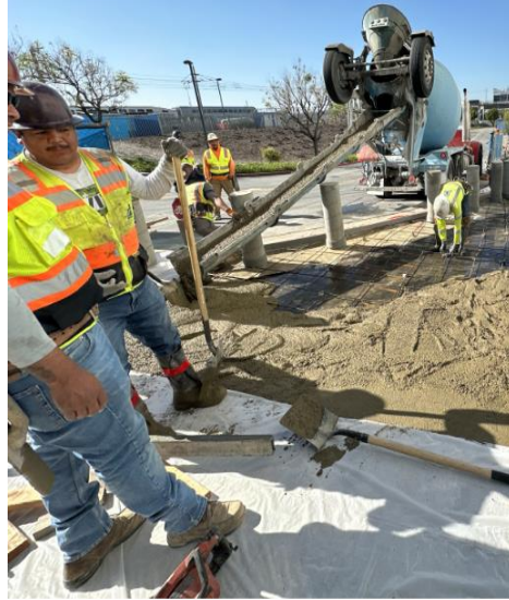
Headquarters Physical Security Upgrades—Exterior Security-Slab Concrete Placement Bollards
