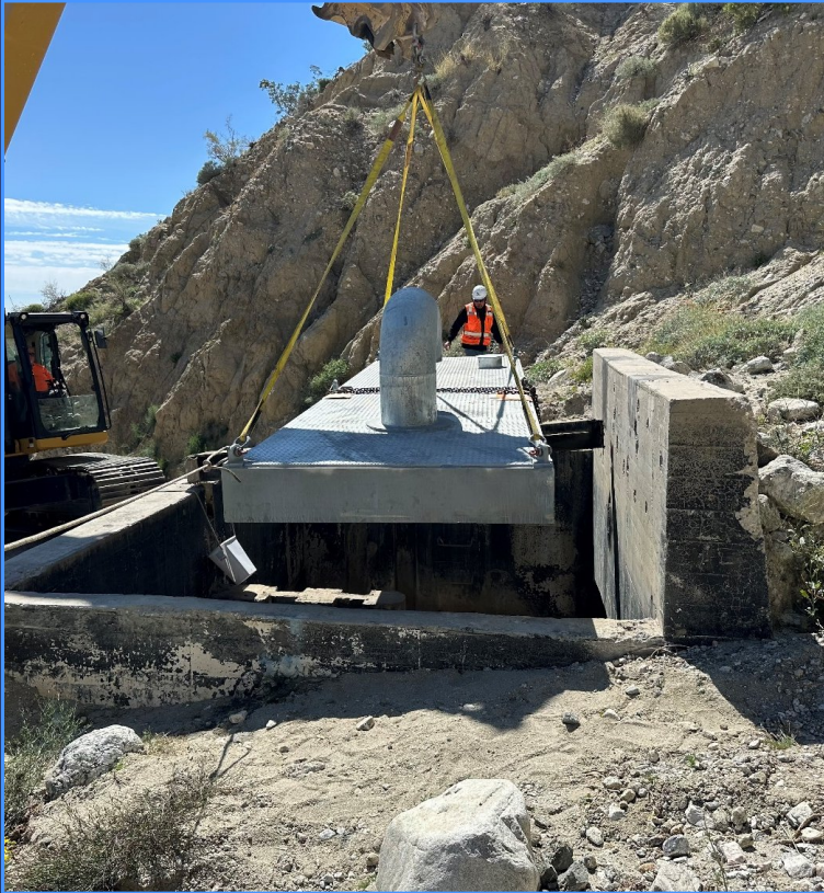
Transition Structure Cover Installation near Desert Hot Springs
