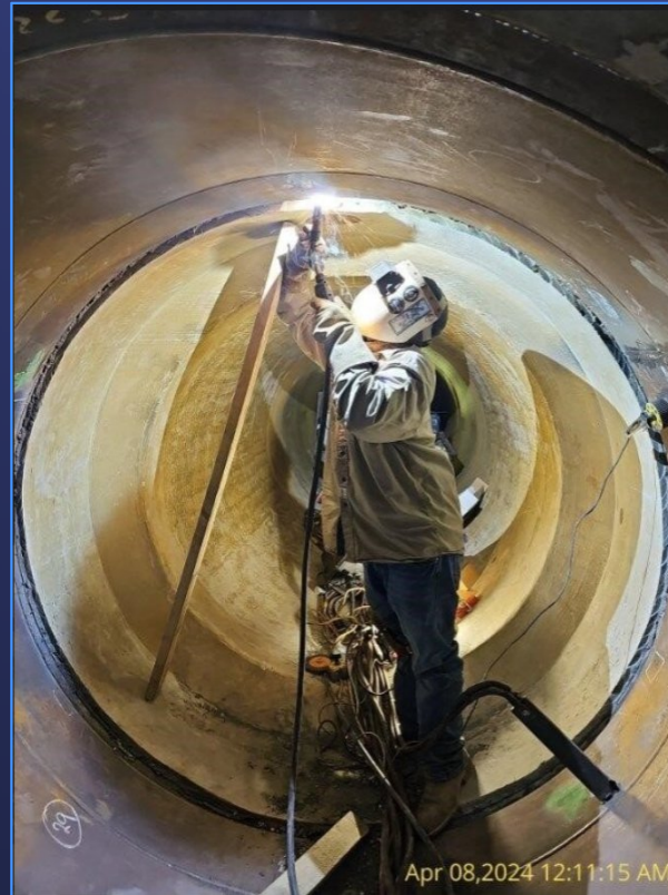
Circumferential Welding of Steel Pipe
