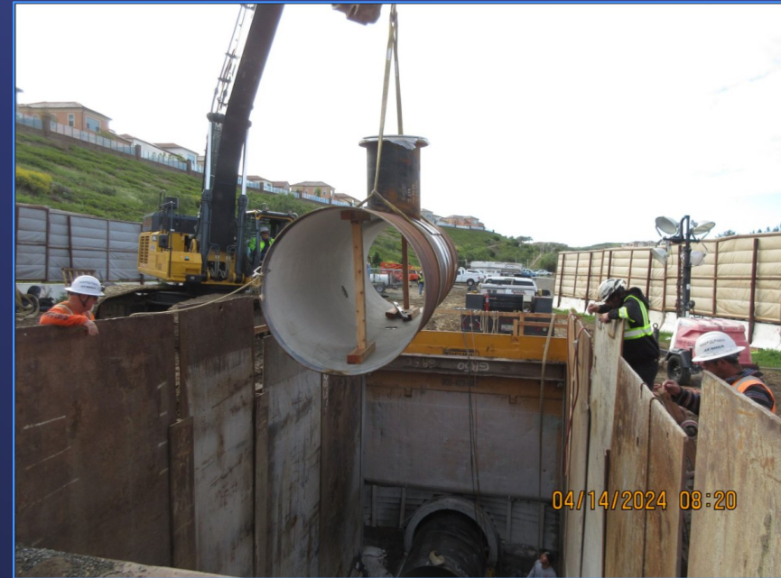
Installation of Closure Pipe
