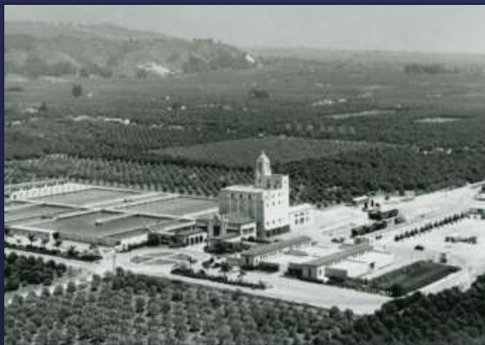
Softening and Filtration Plant, 1940s (Weymouth Plant)
