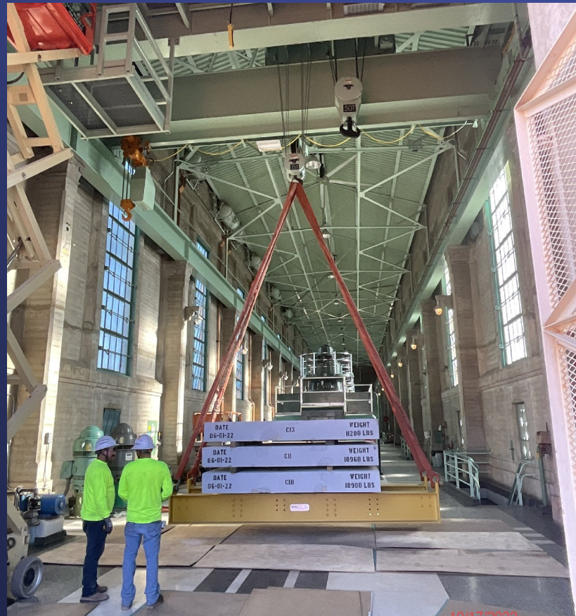
Load Testing New Crane at Gene Pumping Plant
