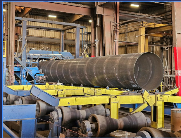
Fabricating Liner Pipe
