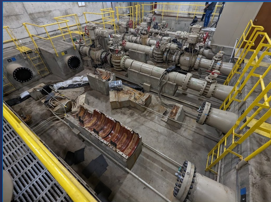
Covina Pressure Control Structure - Valve Replacement
