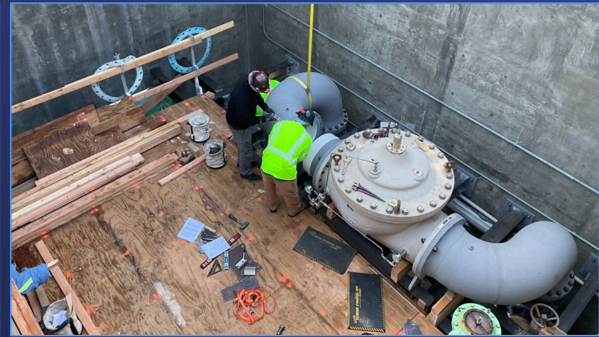
Installing PRV Near OC-88
