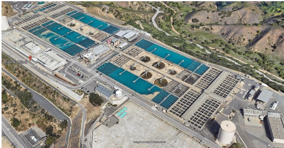
Robert B. Diemer Water Treatment Plant
