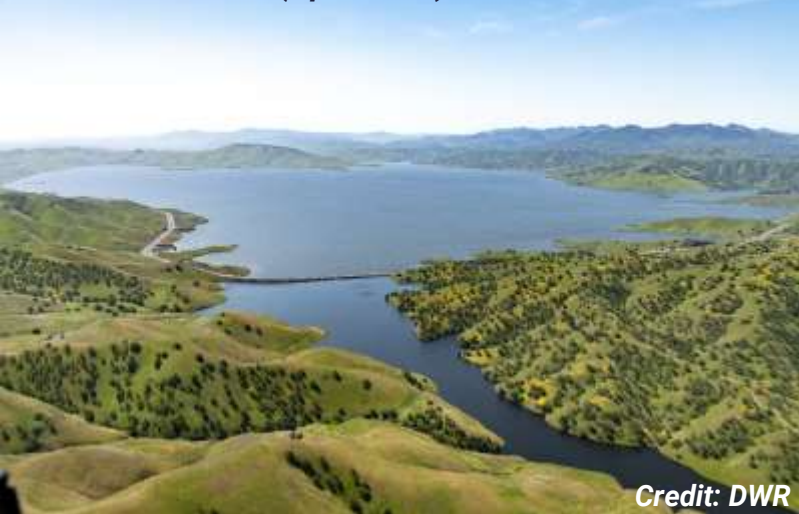
San Luis Reservoir (April 2023)
