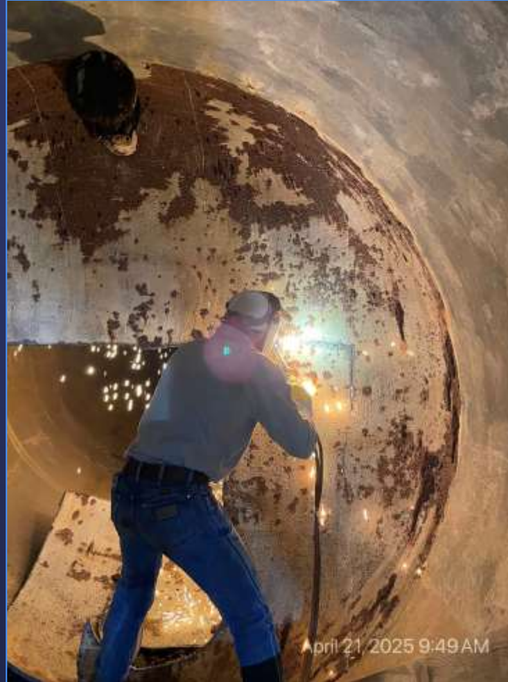
Welder Cutting Bulkhead
