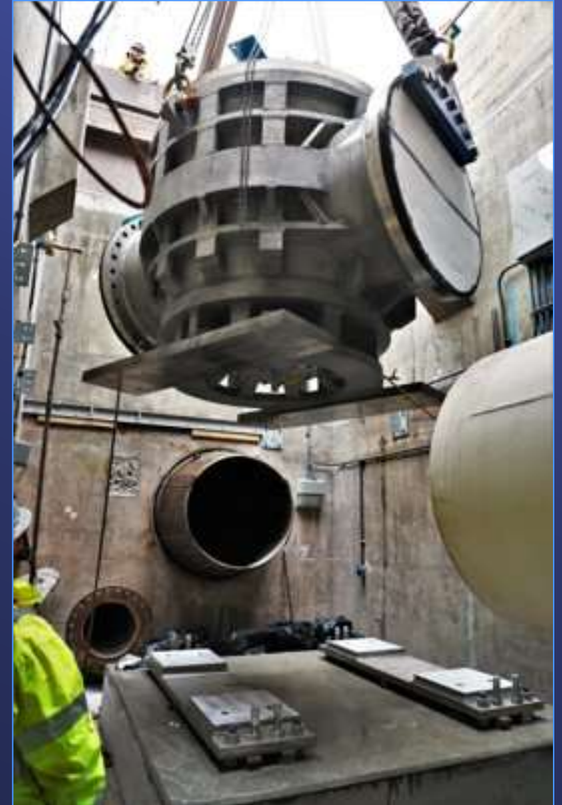
Valve Installation
