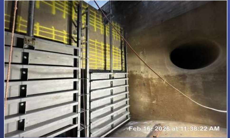
San Jacinto Diversion Structure Slide Gates Replacement
