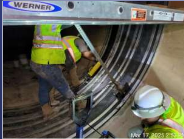
Freda Siphon Internal Bands Installation
