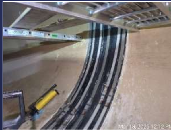
Freda Siphon Internal Bands Installation
