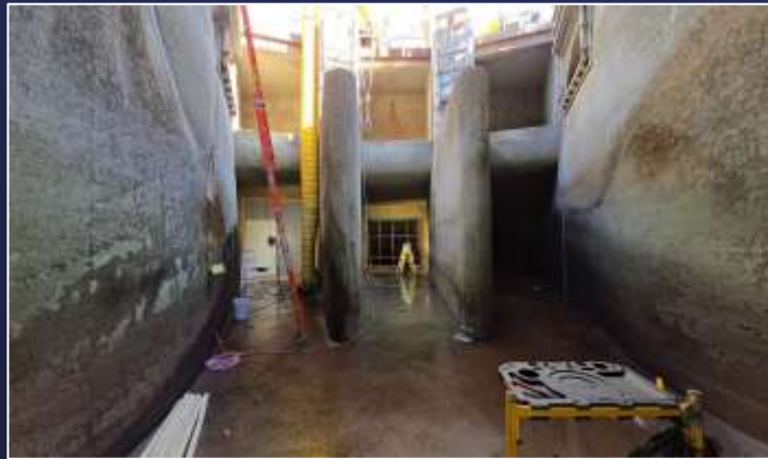
Iron Mtn. Head Gate Inspection
