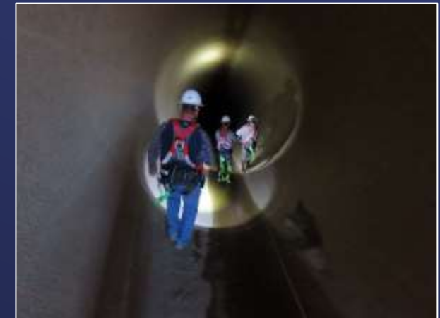
Hinds Inlet Manifold Inspection
