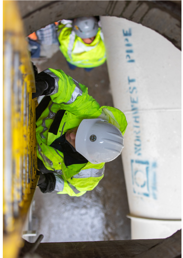
Repairs to the Second Lower Feeder.
