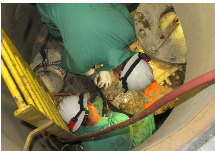
Repairs on the Calabasas Feeder.
