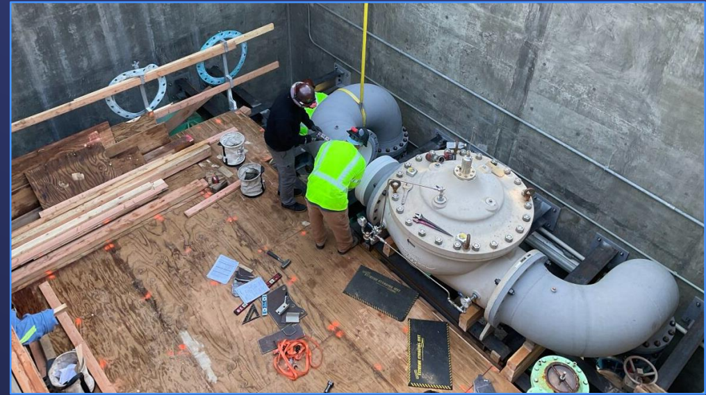
Installing PRV Near OC-88
