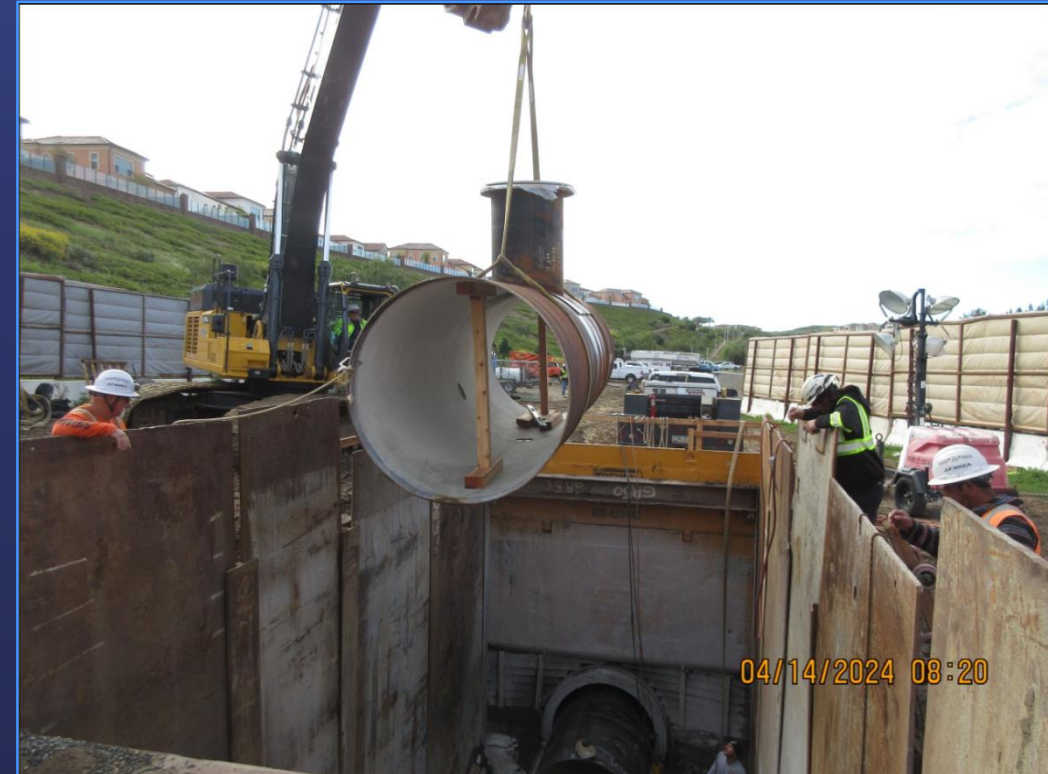
Installation of Closure Pipe
