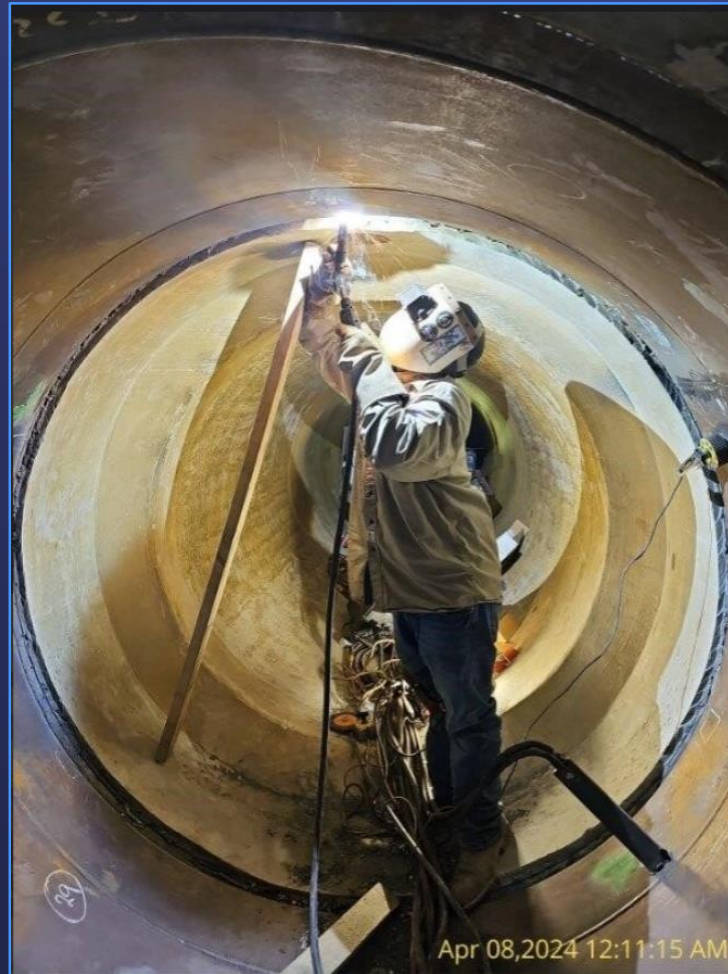
Circumferential Welding of Steel Pipe
