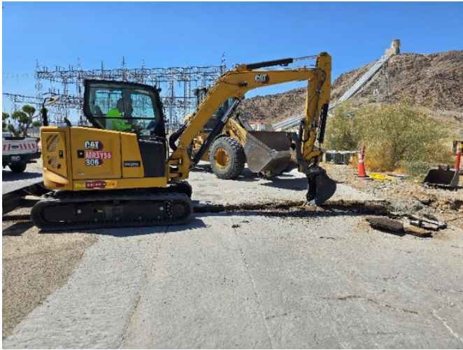
Staff excavating trench at the Eagle Mountain village
