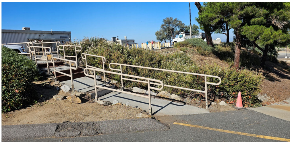
Newly replaced handrails in parking lot at the Skinner plant
