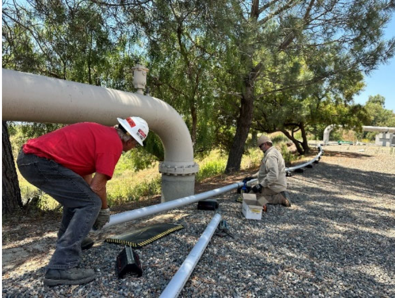
Installing conduit for temporary power at OC-88 pump station
