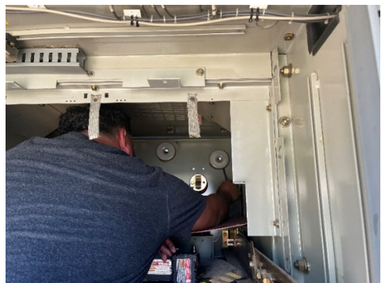
Replacement at OC-88 pump station
