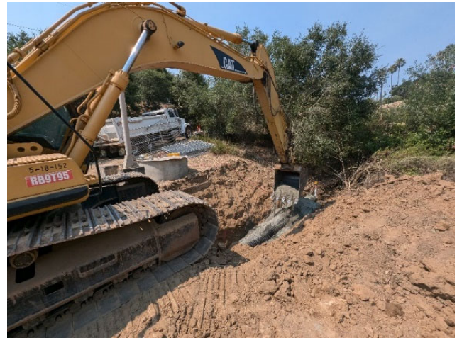
Staff installing new drainage pipe near San Diego Pipeline Nos. 4 and 5
