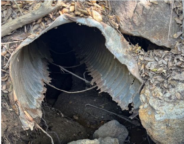
Existing drainage culvert near San Diego Pipeline Nos. 4 and 5
