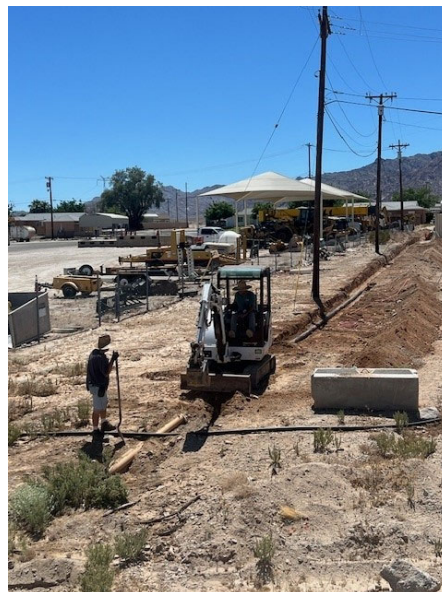
Installation of a new drain line at Iron Mountain
