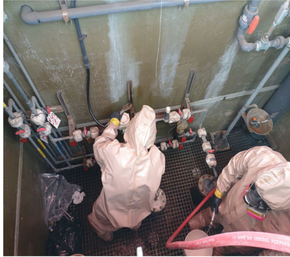
Repairing a fluoride flow meter at the Weymouth plant
