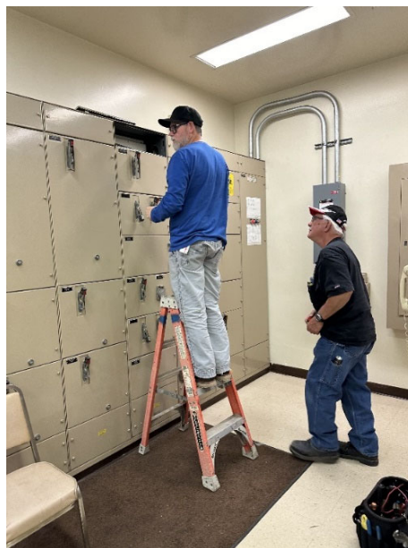
Electricians verifying cable sizes in electrical equipment at San Dimas HEP
