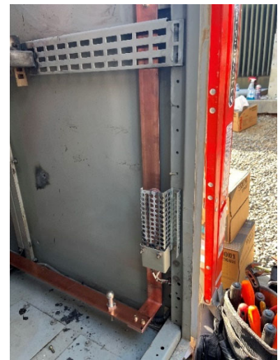
Installation of new buss
