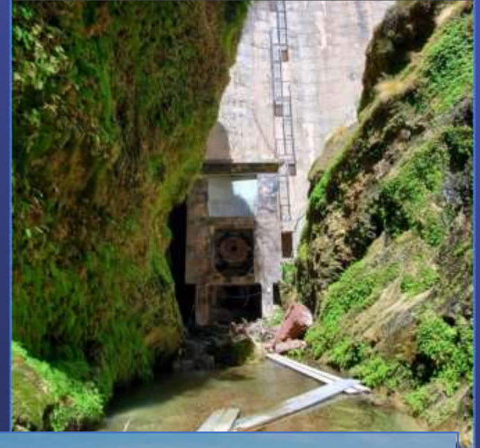
Copper Basin Discharge Structure
