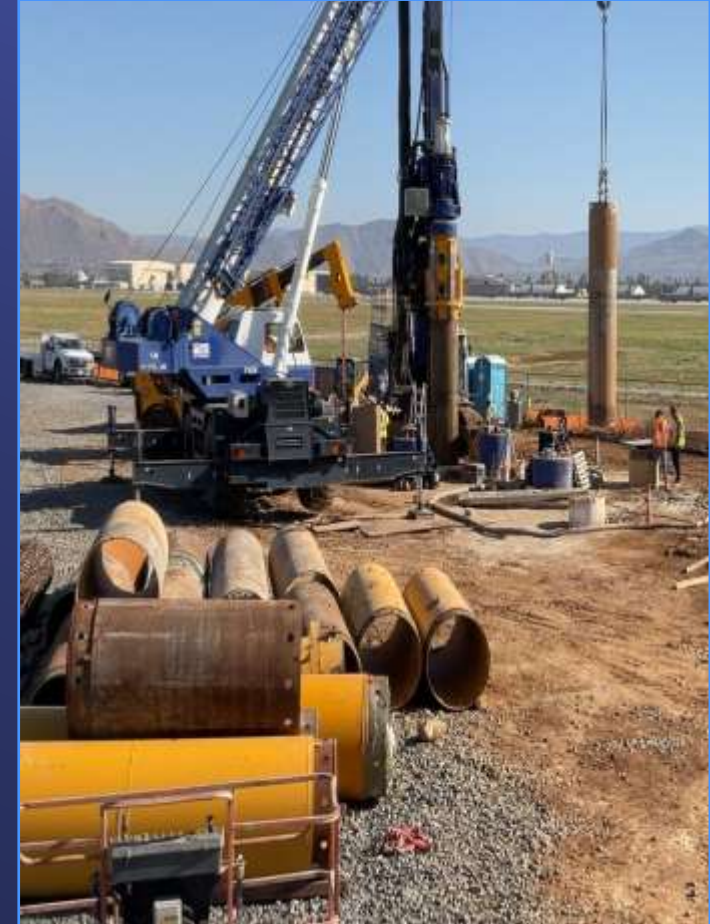
Contractor drilling shaft piles
