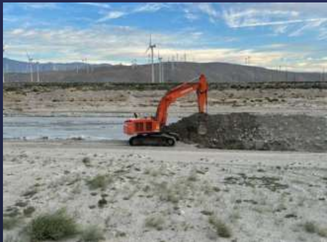
Repairing Whitewater Conveyance Channel
