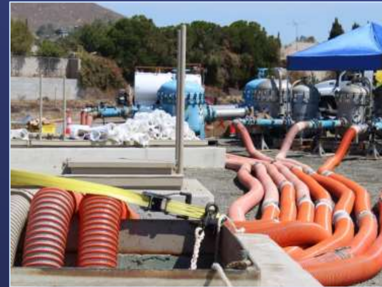
Quagga mussel filtration for pipeline dewatering
