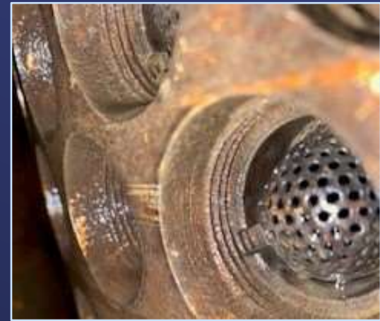
Jensen Plant Ozone Cooling System Strainer
