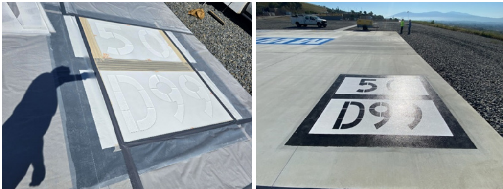
Application of stencil (left) and completed weight/rotor diameter marking (right)
