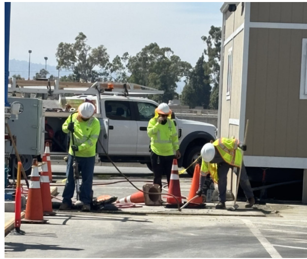
Staff installing a new potable water line for an office trailer at the Napolitano Innovation Center
