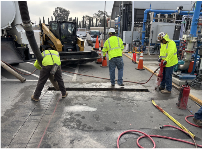
Staff installing a new potable water line for an office trailer at the Napolitano Innovation Center
