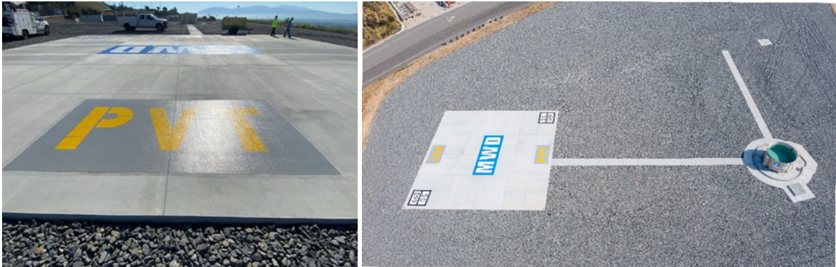
Ground view (left) and overhead view (right) of completed markings for Diemer Heli-pad
