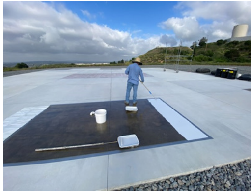
Site prep of concrete pad prior to coating application
