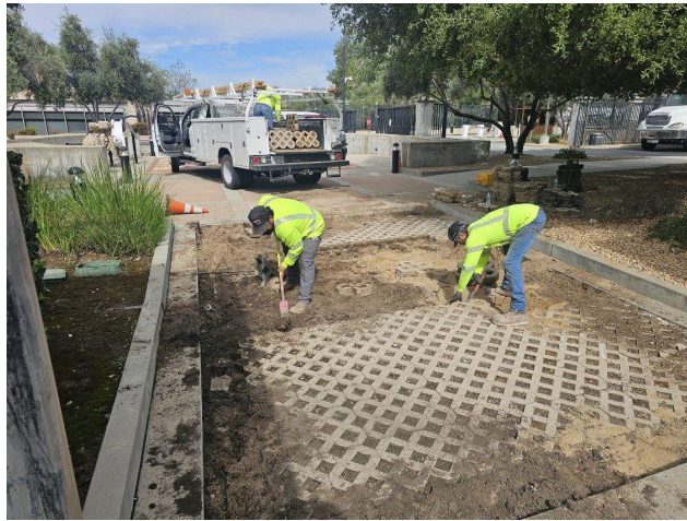
Staff removing pavers within a walkway at the La Verne facility
