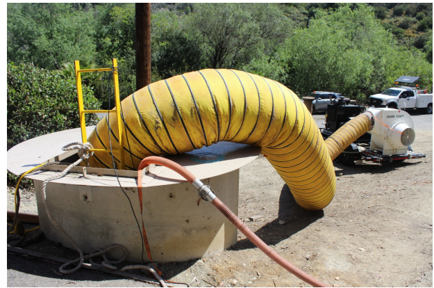
Inspection team preparing for entry into the Irvine Cross Feeder (left) and ventilation setup to allow staff to inspect the feeder (right)
