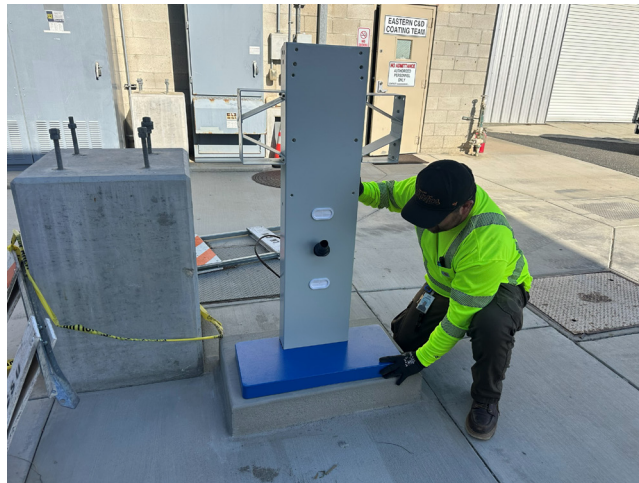
Staff installing a new electric vehicle charger base at Lake Mathews
