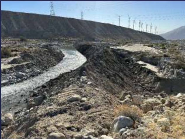
Whitewater Channel Repair
