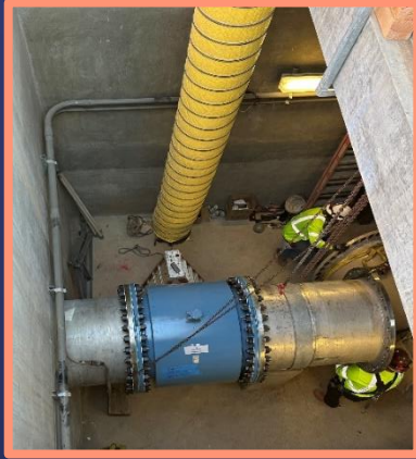
EM-24 Flowmeter Replacement Shutdown
