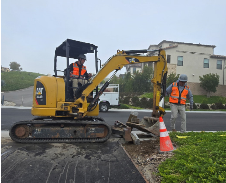
Allen-McColloch Pipeline Urgent Relining —Removing the Existing Sidewalk
