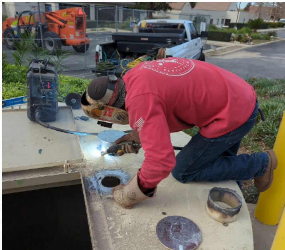
Rialto Pipeline Rehabilitation – Welding of Valve Stem Cap at CB-11
