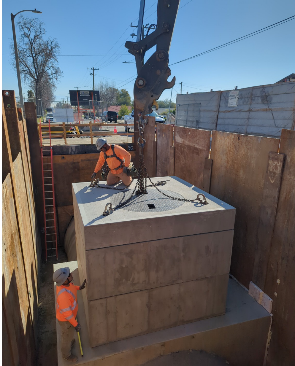
Rialto Pipeline Rehabilitation – Installation of Access Structure
