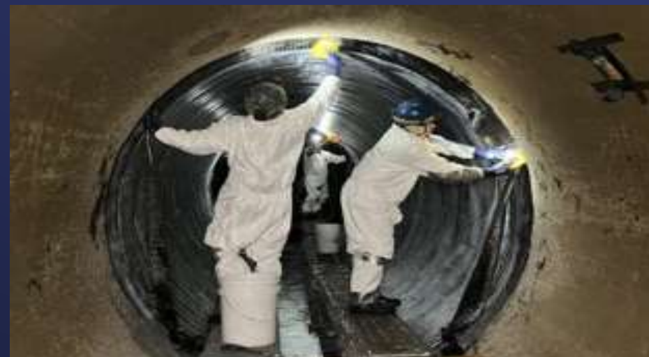
Sepulveda Feeder Carbon Fiber Lining
