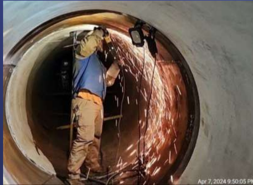
Welding new steel liner pipe
