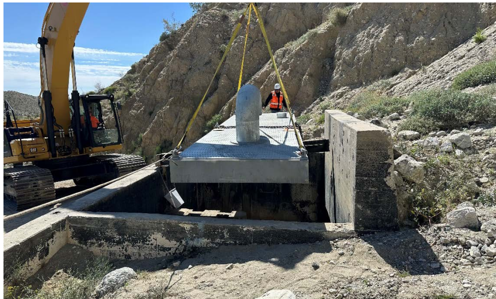
Transition Structure Cover Installation at Site 23 east of Hinds Pumping Plant near Desert Hot Springs
