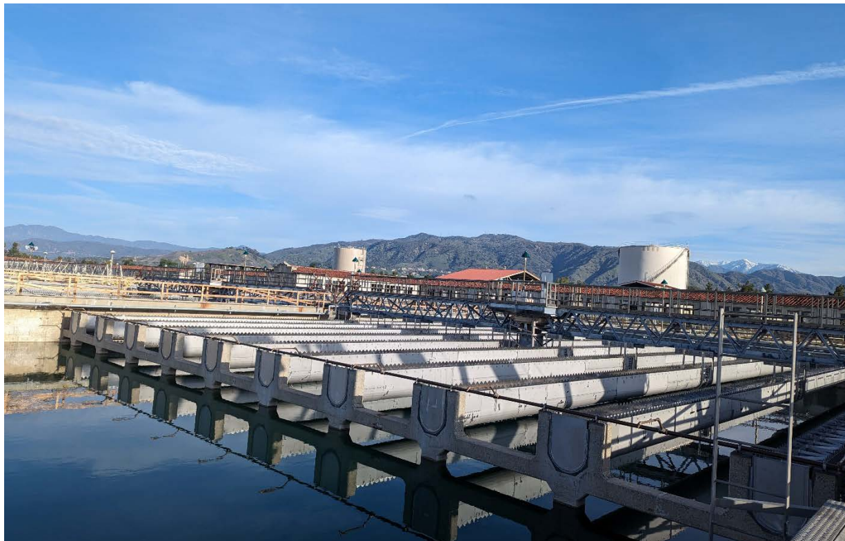
New stainless-steel launders in Basin No. 8
