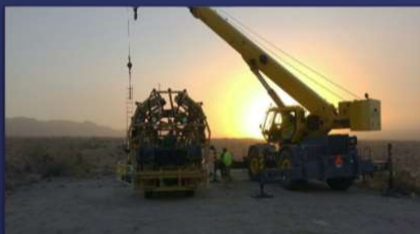
Colorado River Aqueduct
