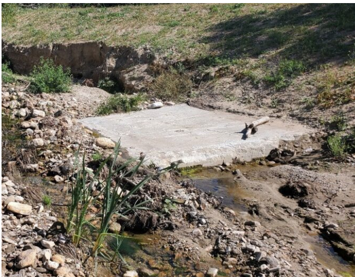
Exposed West Valley Feeder No. 2 (left) and staff installing riprap grade control (right)
