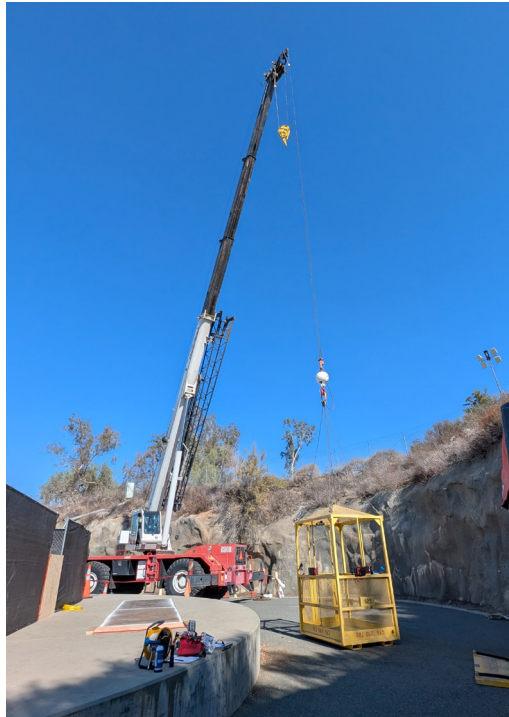
Main entrance to the shaft and tunnel system at Lake Mathews being lowered down 160 feet by crane
