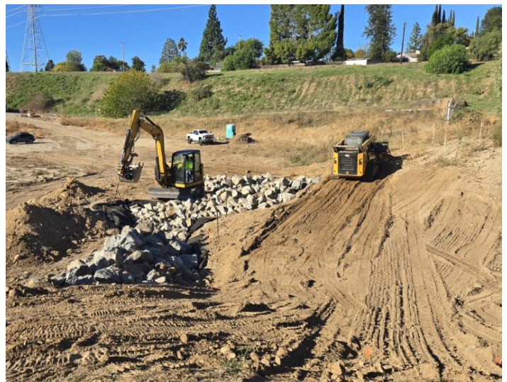
Exposed West Valley Feeder No. 2 (left) and staff installing riprap grade control (right)
