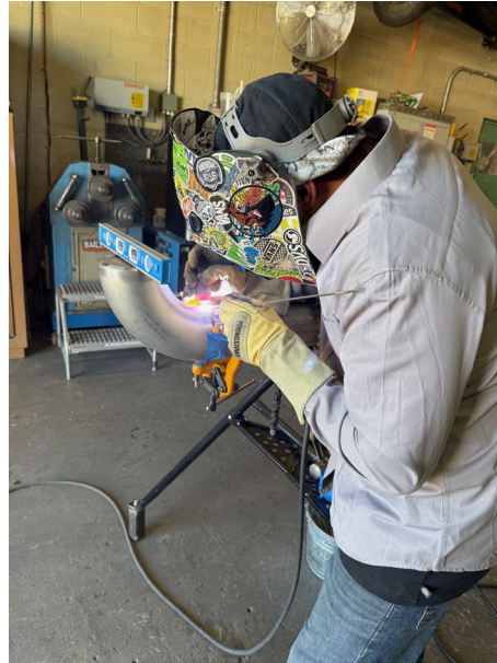
Staff fabricating stainless pipe for Hinds pump plant Unit 5 cooling water system
