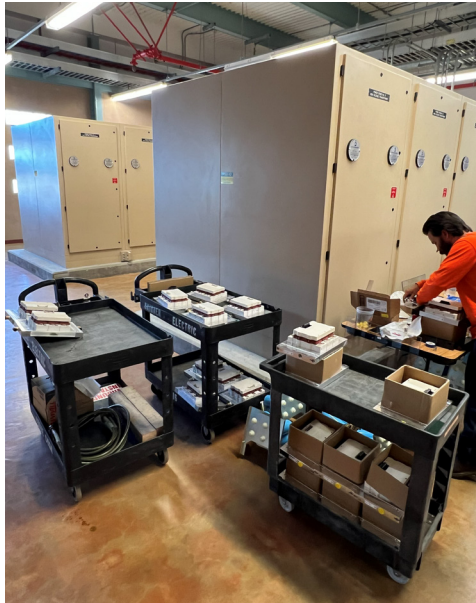
Skinner staff staging ozone generator components for replacement
