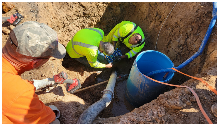
Staff repairing a cooling water pipeline leak at Iron Mountain pump plant
