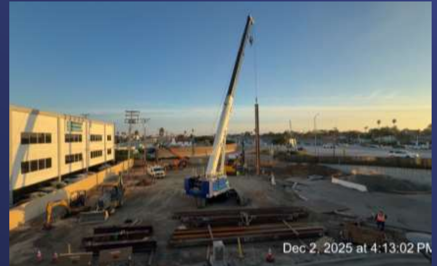
Sepulveda Feeder Pump Stations Stage 1 Venice Pump Station Construction
