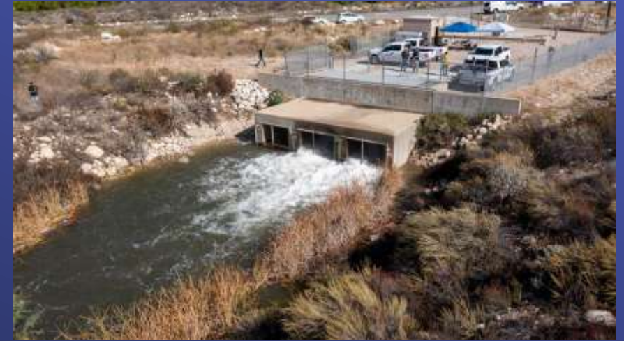
Pumped Flow Delivered to SBVMWD's Facility from Successful Pump Test in Oct 2025
