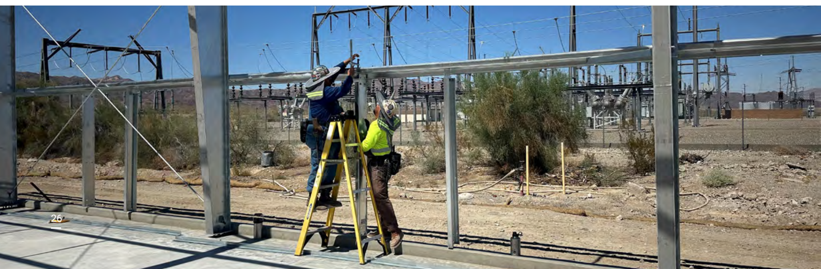
Iron workers installing CRA storage building framing at Eagle Mountain
