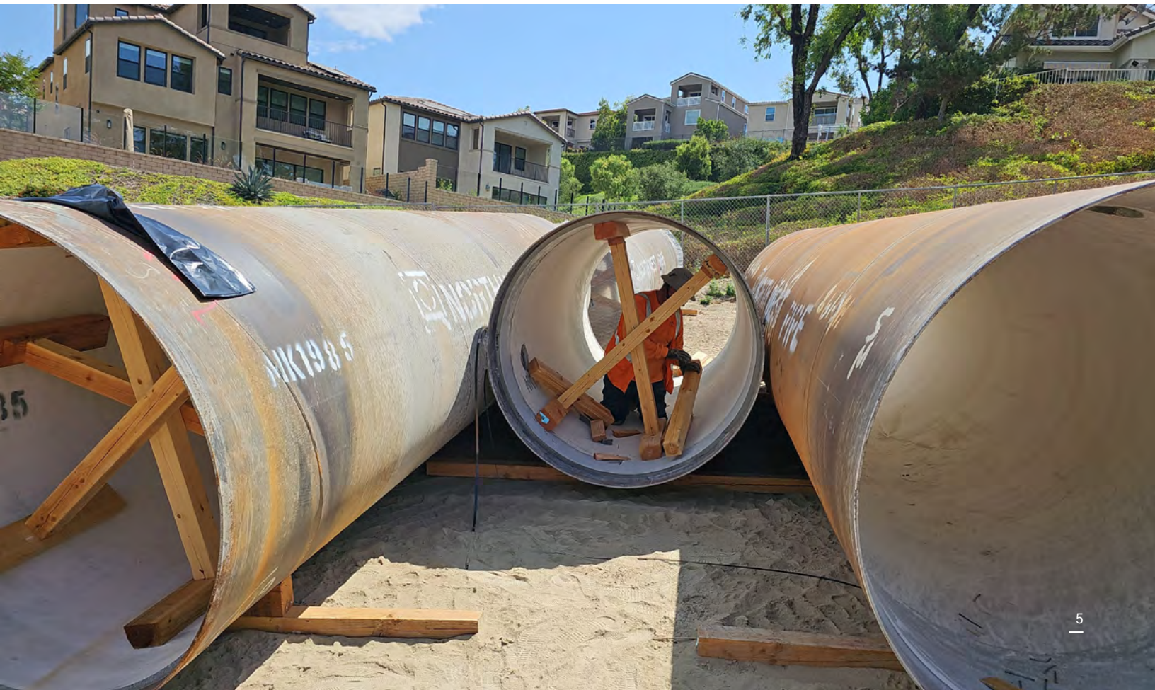
Welded steel pipe used for the Allen McColloch PCCP Urgent Rehabilitation
