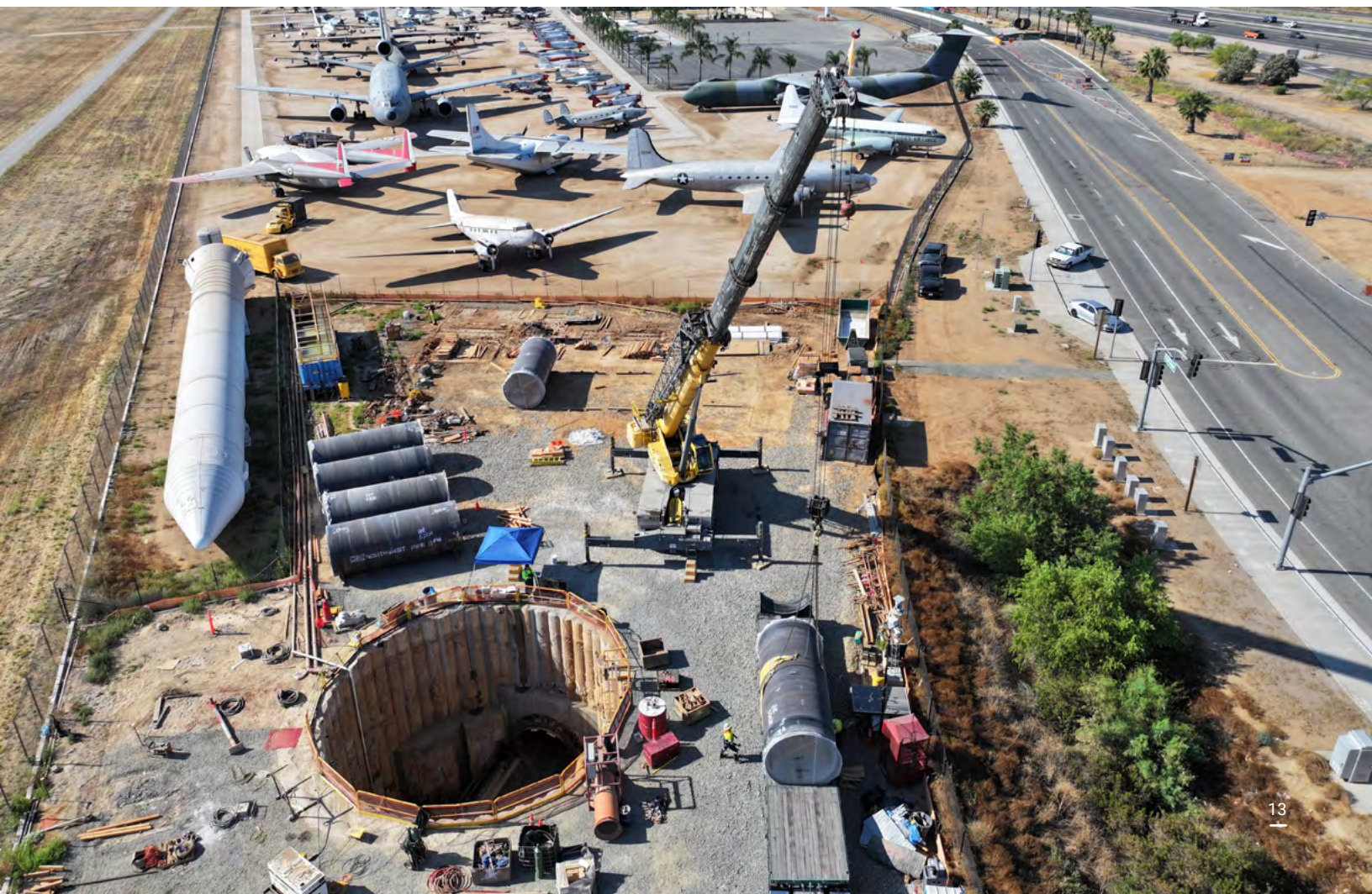
Shaft for Perris Valley Pipeline I-215 Crossing near March Air Reserve Base
