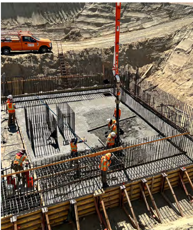
Valve vault foundation for Badlands Tunnel Project
