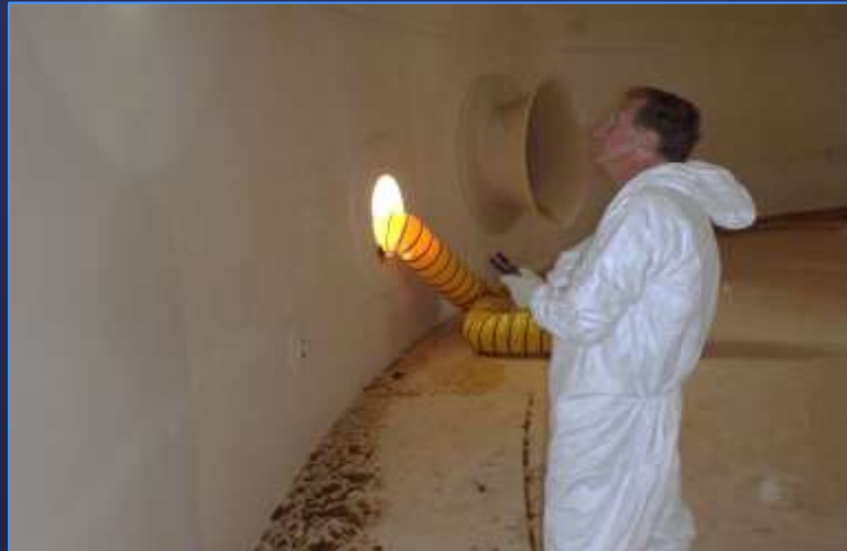
Tank Lining Inspection
