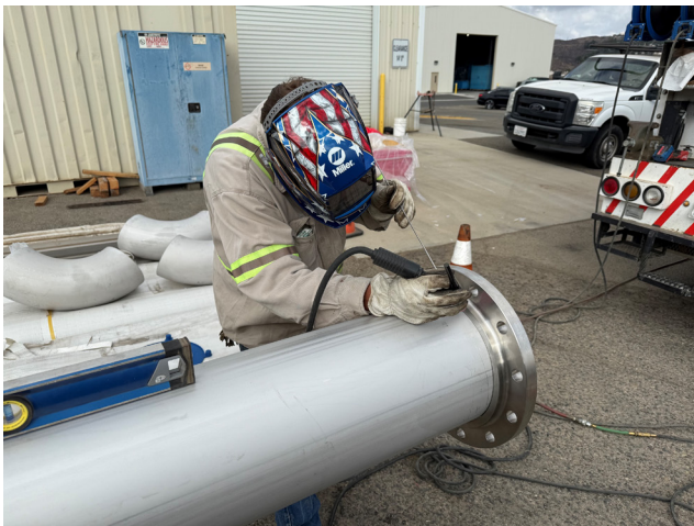
Staff welding stainless-steel piping
