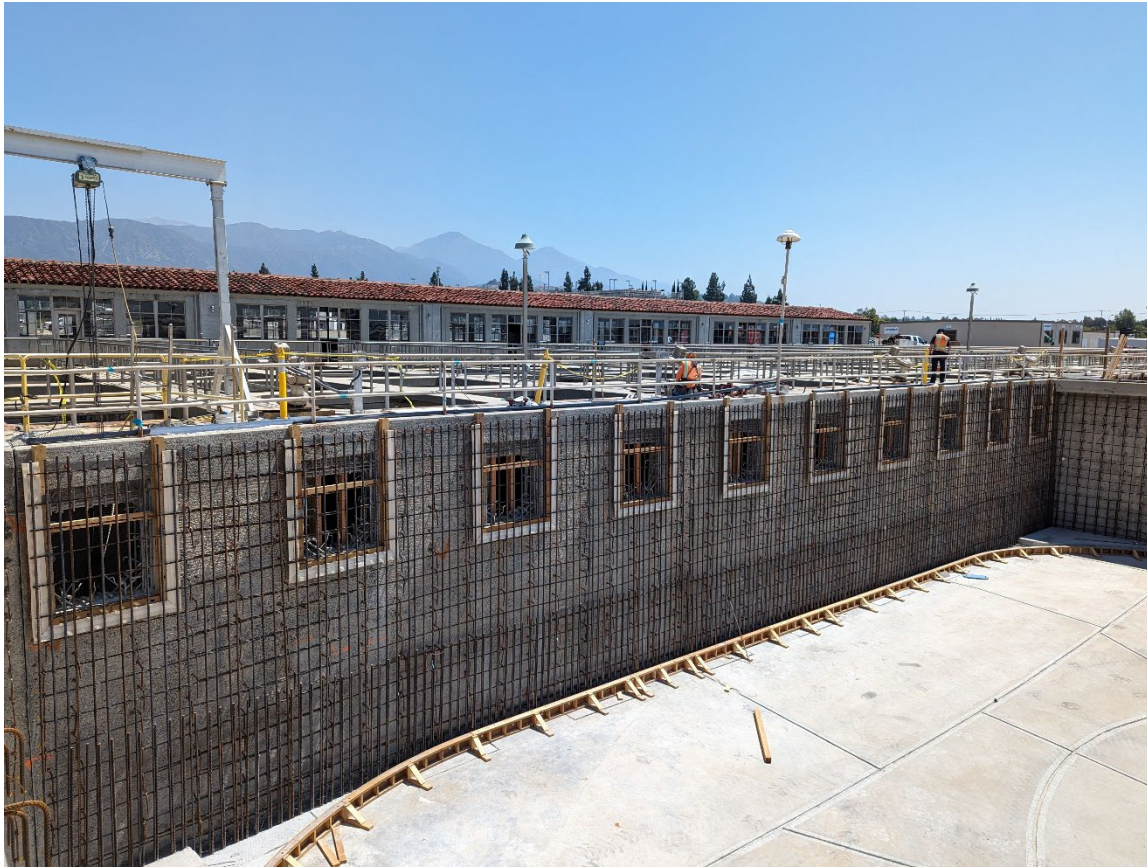
Figure 4-1: Seismic Reinforcement of Weymouth Basin 7
