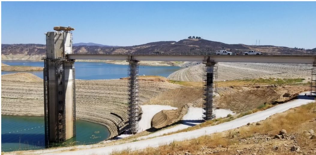
Figure 8-1: Castaic Dam High Tower and Access Bridge, with scaffolding installed for installation of carbon-fiber reinforced polymer wrap on piers
