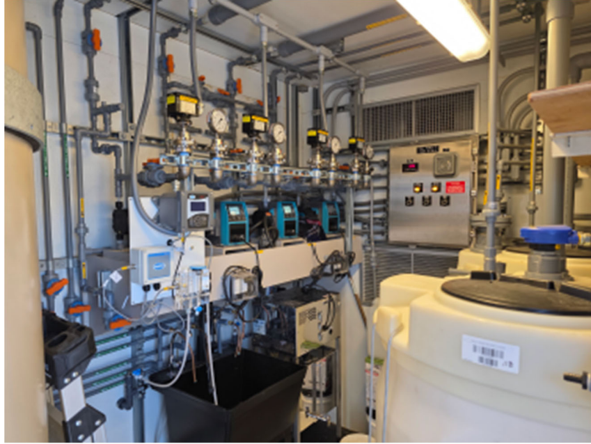
CRA Domestic Water Treatment System — Temporary Skid Commissioning
