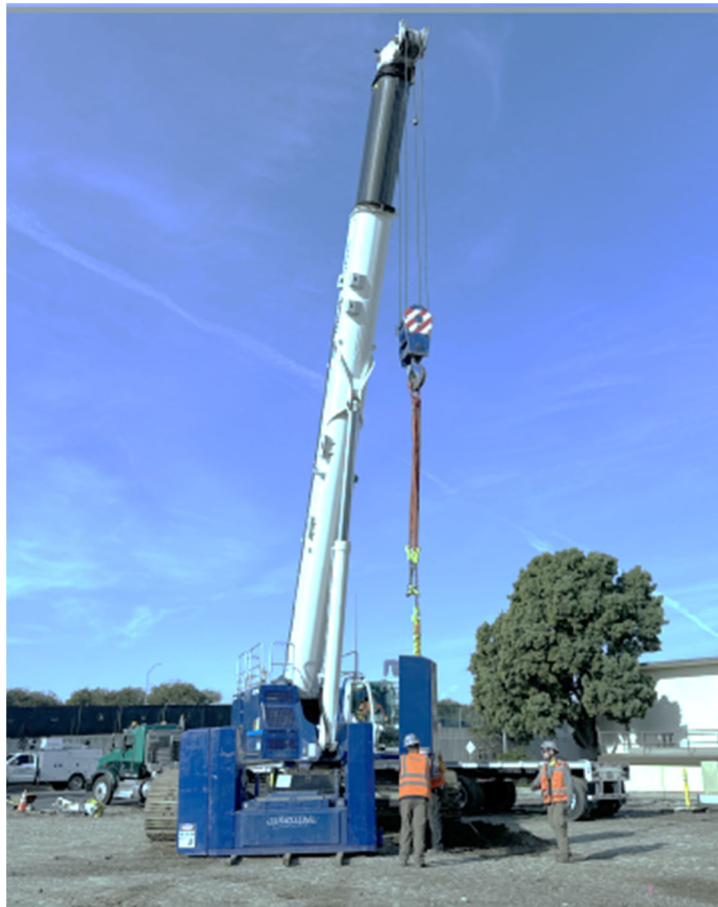
Sepulveda Feeder Pump Stations — Venice PCS Contractor J.F. Shea Assembling Crane Counterweights
