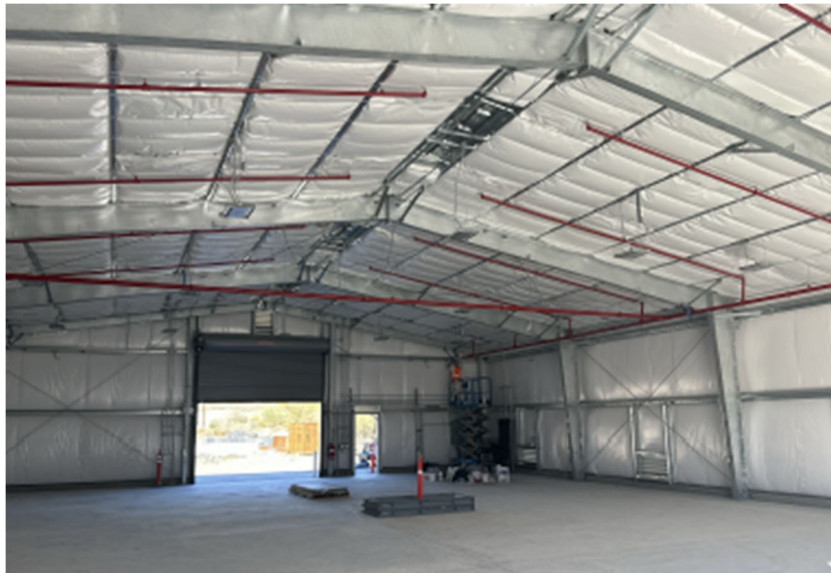
CRA New Storage Buildings — Eagle Mountain Maintenance Storage Building Techno Crew Coating (Red Paint) fire Sprinkler Pipe
