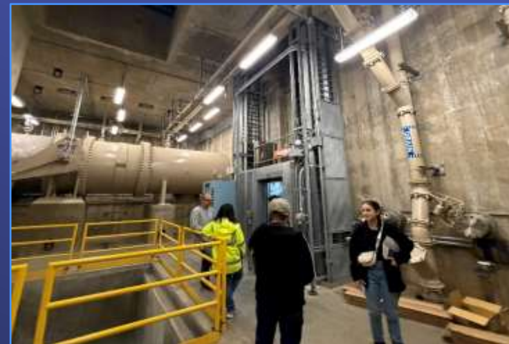
Diamond Valley Lake I/O Tower
