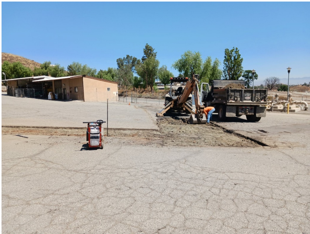
Preparing subgrade for paving over the newly installed sewer line near Lake Mathews Building 6
