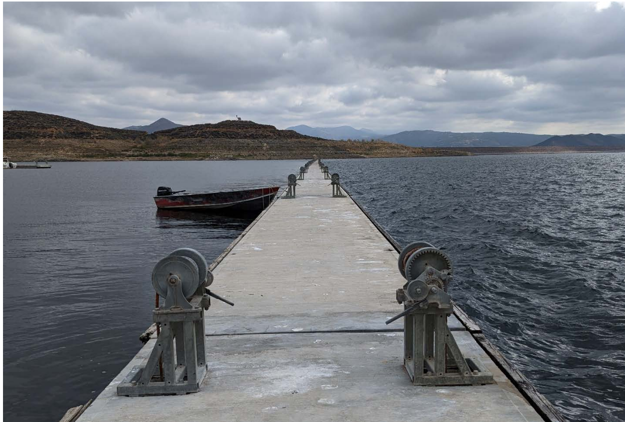
Existing floating wave attenuator at Diamond Valley Lake: Looking from West to East
