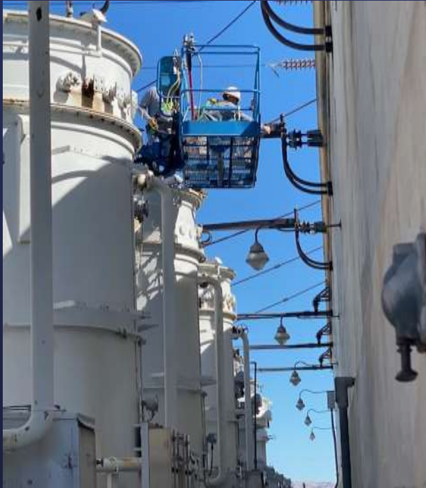
230kV Transformer
