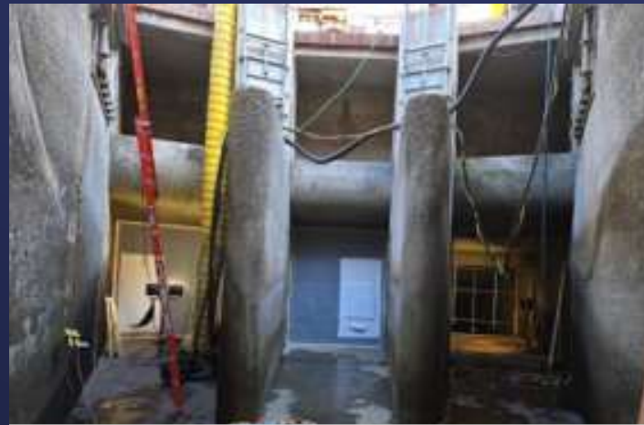
Iron Mtn Head Gate #3 Repair
