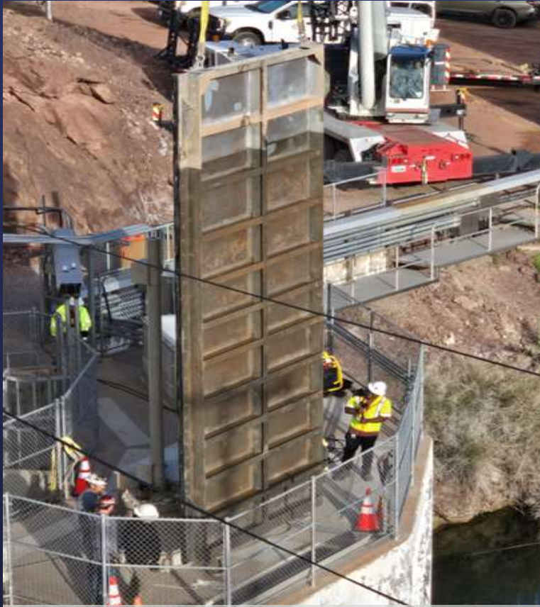
Copper Basin Gate #3 Repair
