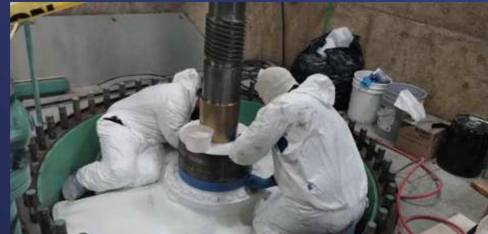
Hinds Unit #4 Discharge Valve Repair
