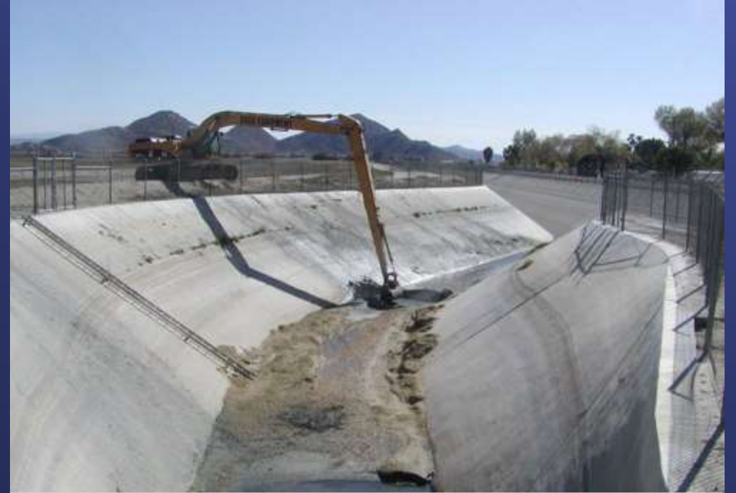
San Diego Canal Cleaning
