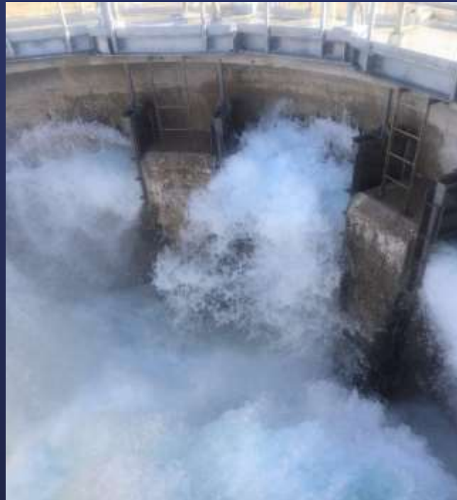
Surge Chamber Flow
