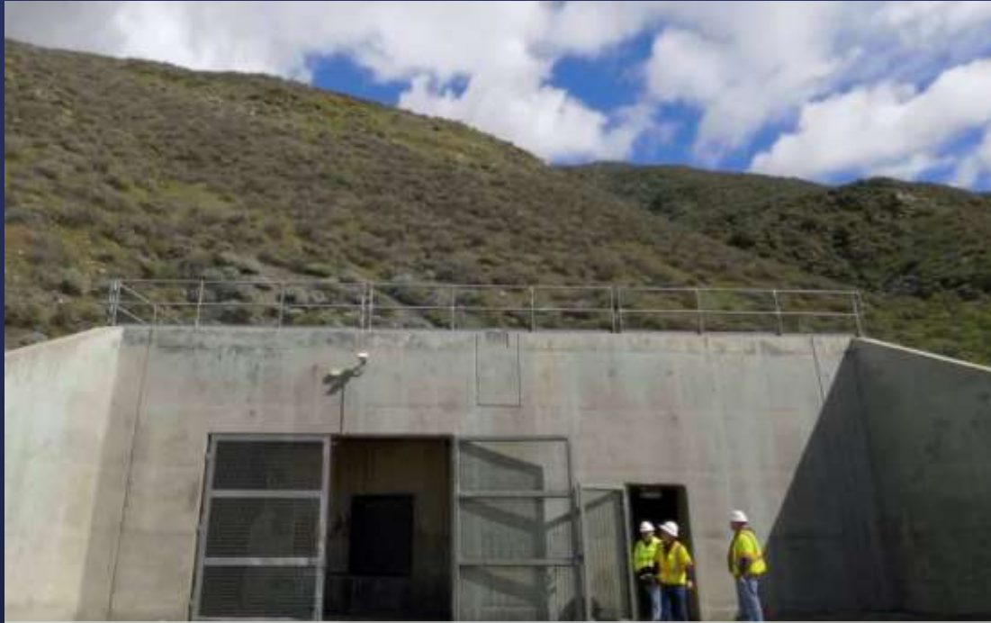
West Portal – San Jacinto Tunnel
