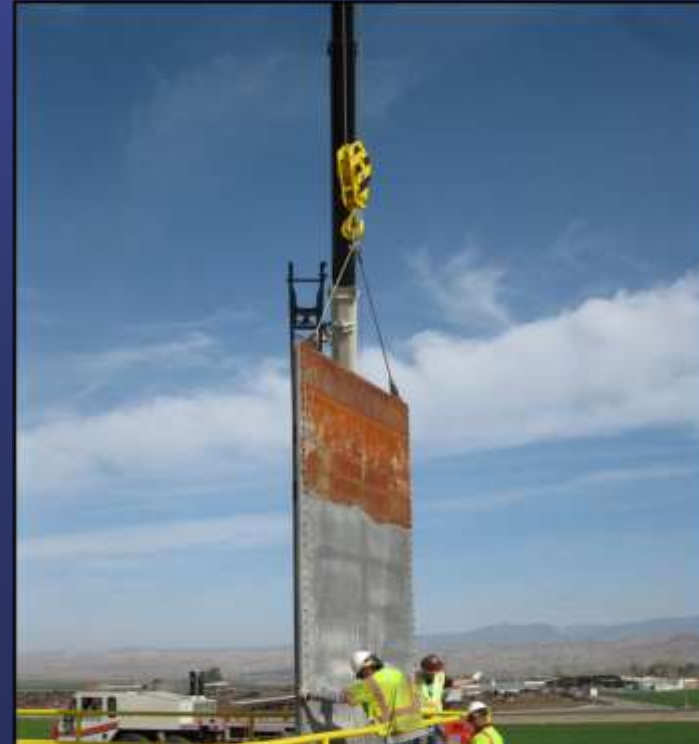
Blocking Gate Installation
