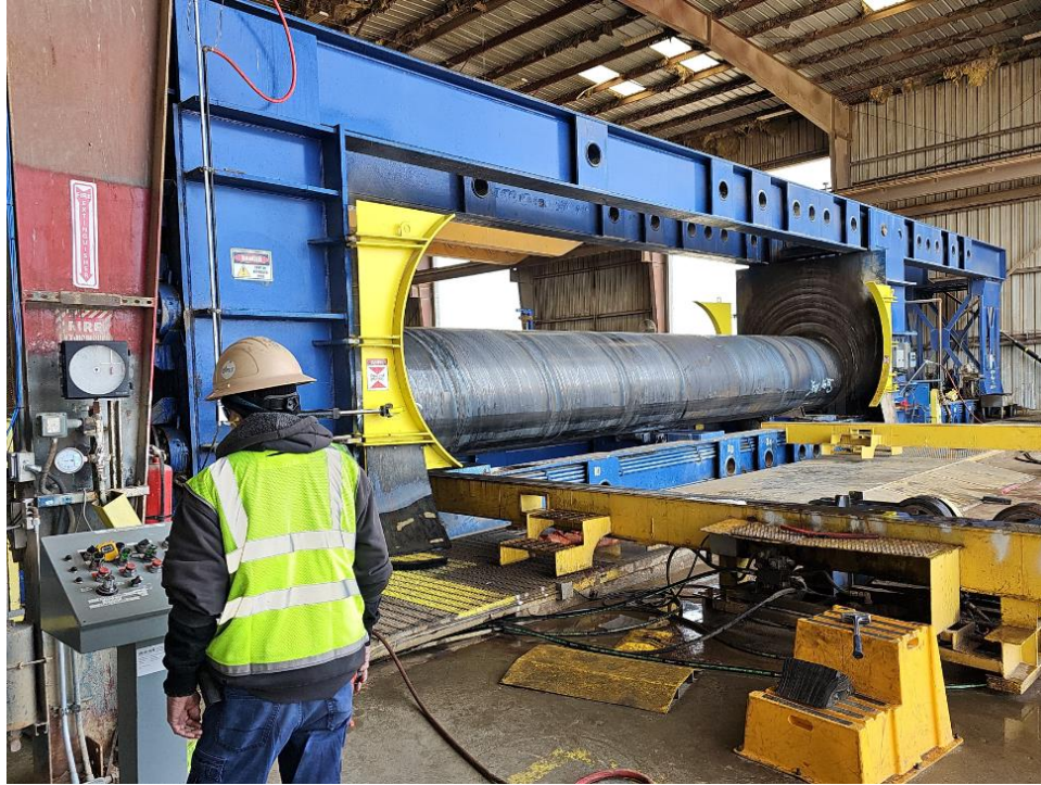
AMP Urgent PCCP Rehabilitation – Hydrostatic testing of 63-inch diameter steel liner pipe
