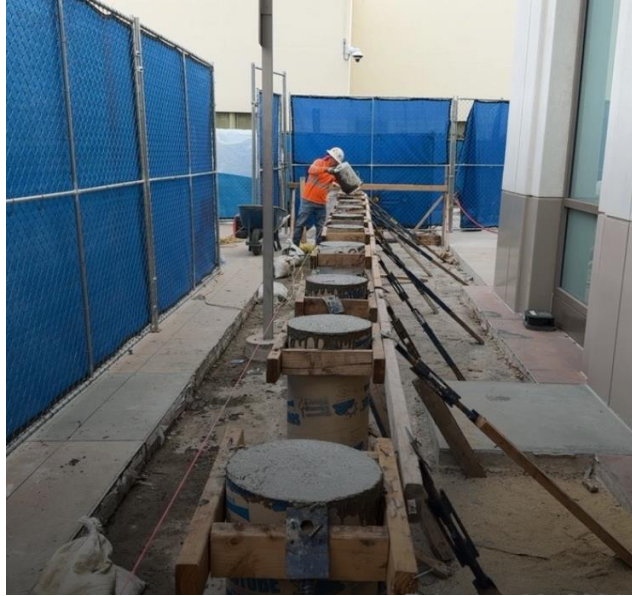
Headquarters Physical Security Upgrades – Installation of bollards
