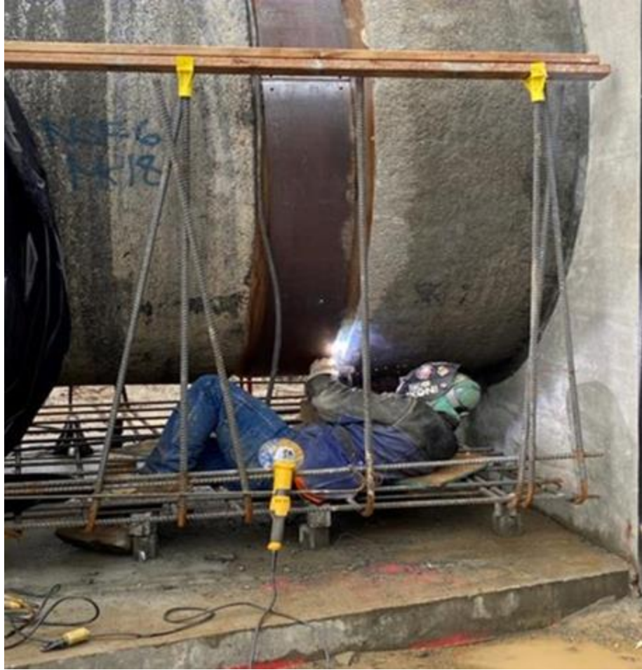
Wadsworth Pumping Plant Bypass – Welding buttstrap
