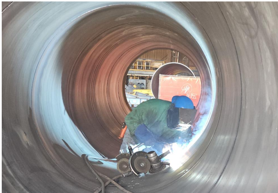
AMP Urgent PCCP Rehabilitation – Welding 60-inch diameter steel liner
