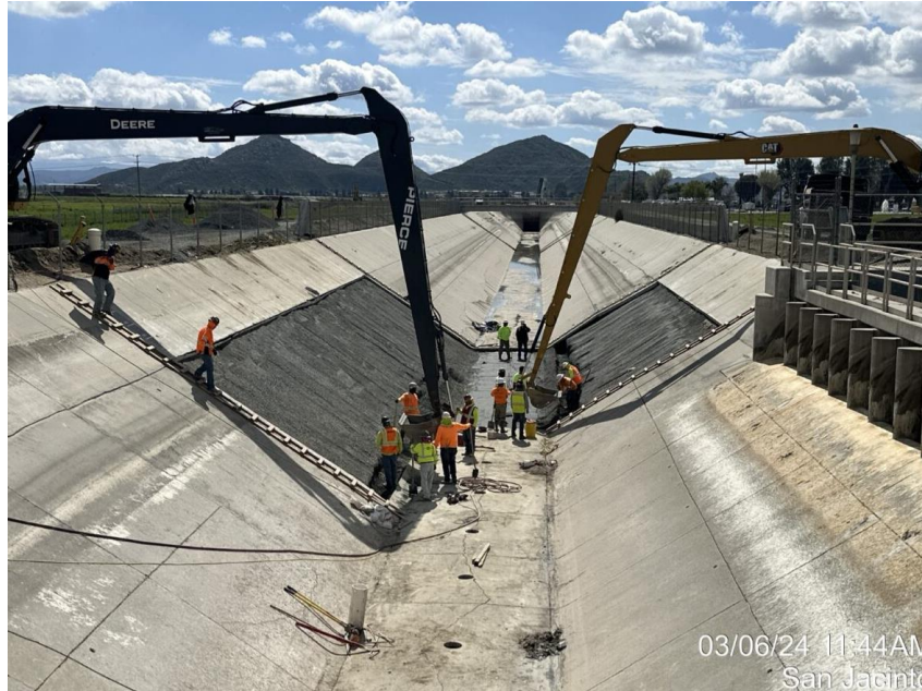
San Diego Canal Relining – Preparation of subgrade prior to concrete placement
