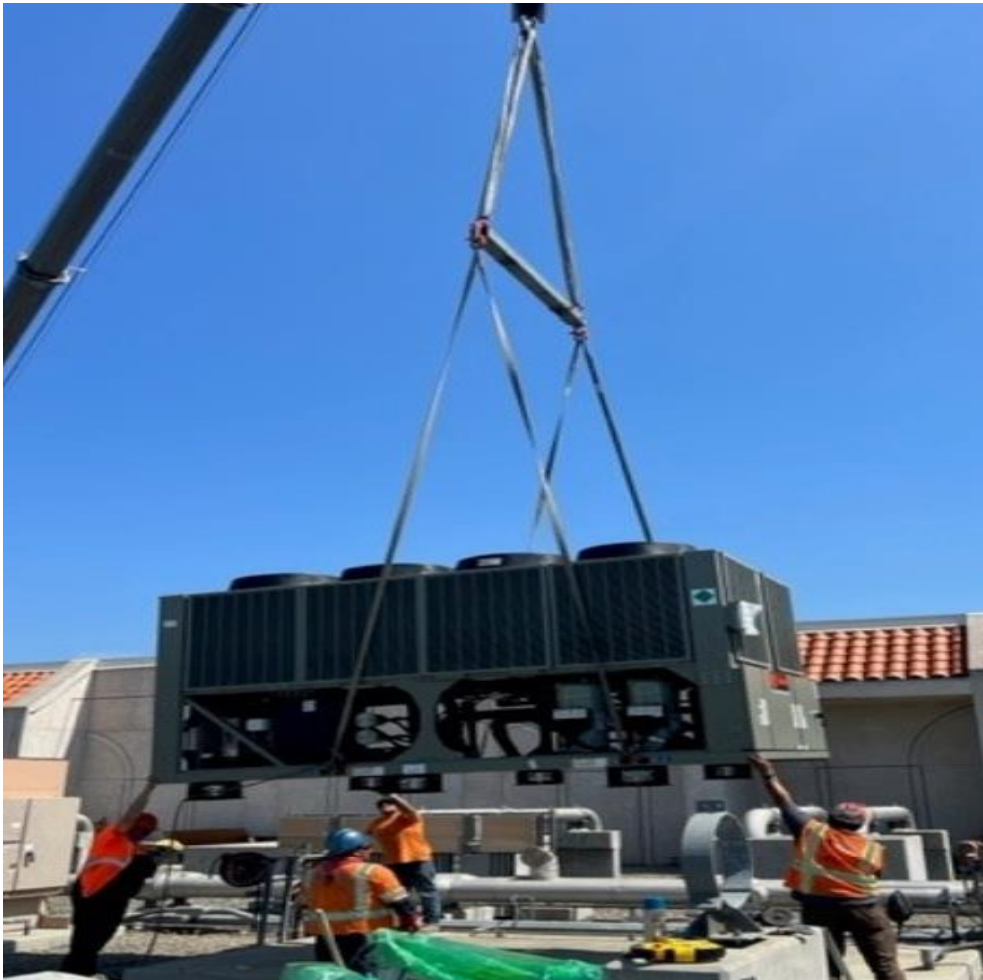
Service Connection OC-88 Chiller Replacement – Chiller installation
