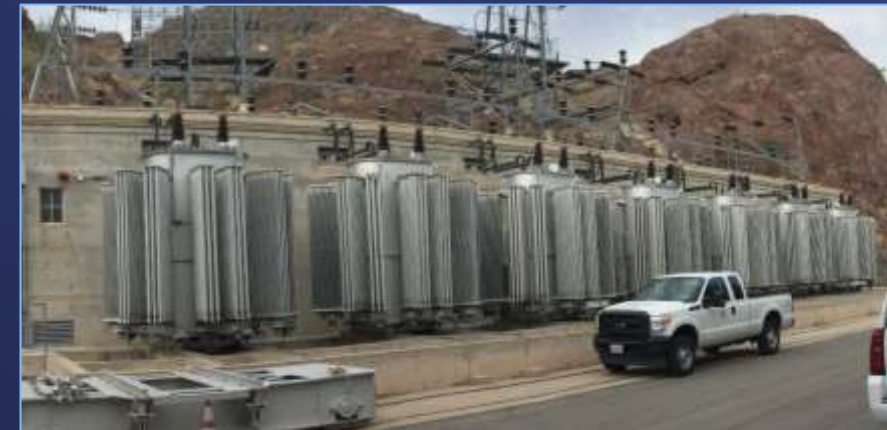
Intake Pumping Plant
