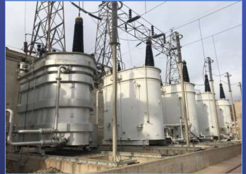
Gene Pumping Plant
