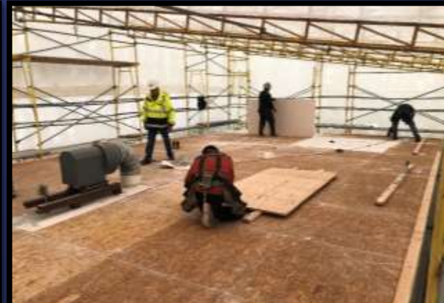
Operations Trailer Roof Replacement
