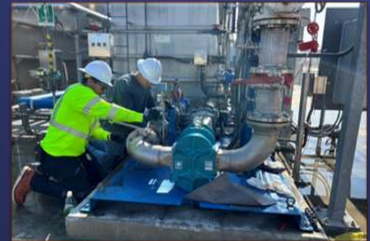
MBR Filtrate Pump Replacement
