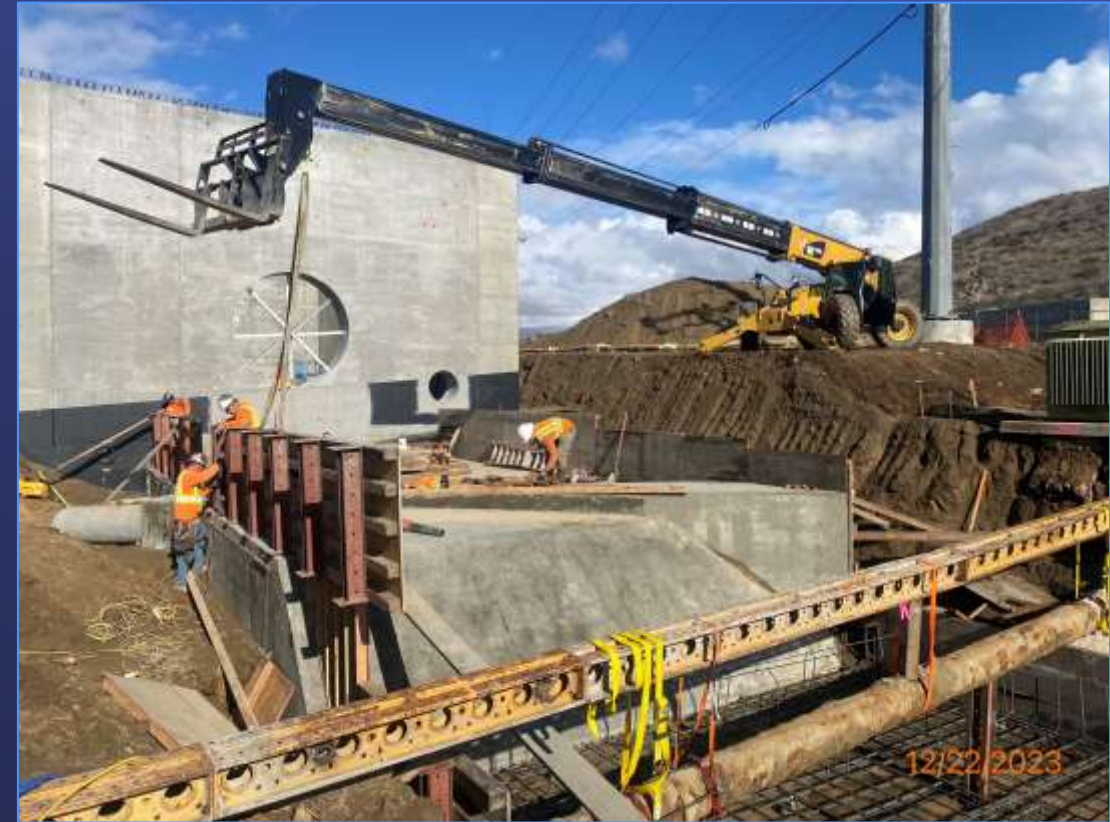
New Vault Structure at Wadsworth Power Plant
