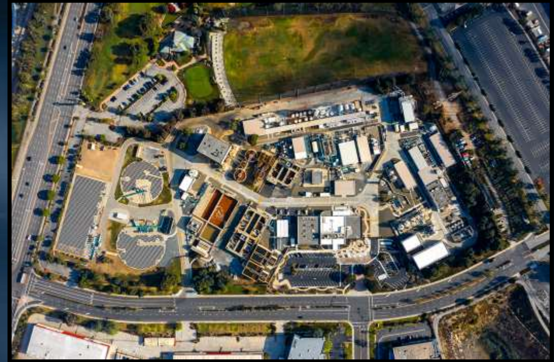
West Basin MWD – Edward C. Little WTP
