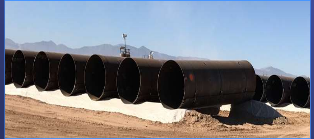
Storage Site with Steel Pipe Liners
