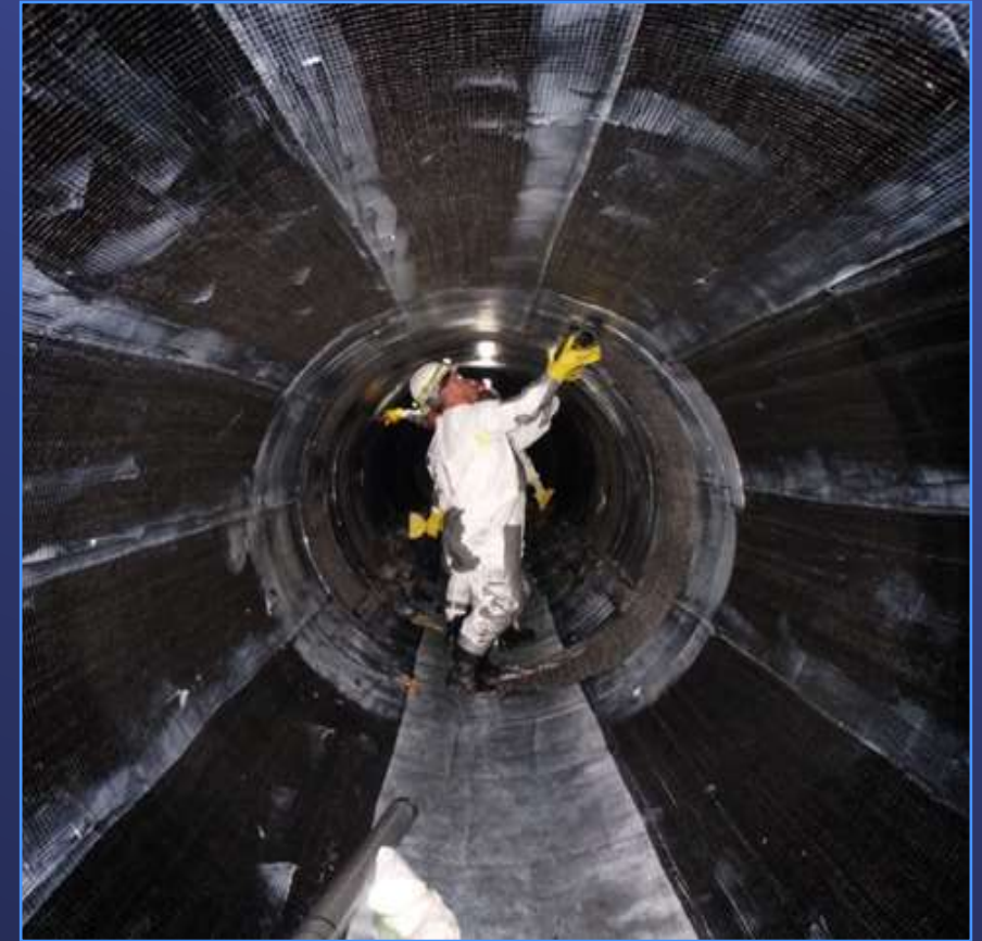
Previous Carbon Fiber Repair Second Lower Feeder
