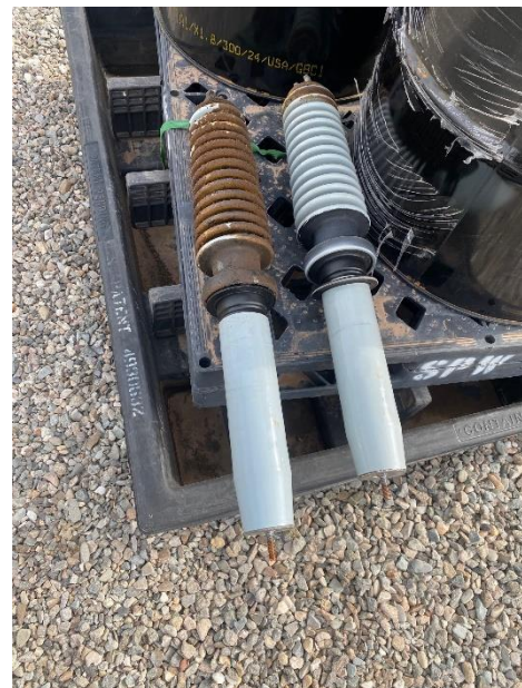
Gene-Peddler Line electrical testing and bushing replacement
