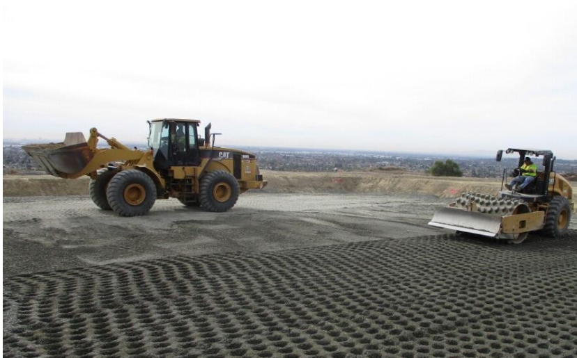
Staff compacting base rock for the helipad at the Diemer plant
