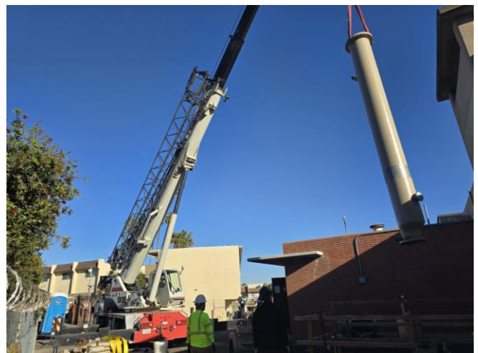
Staff dismantling pipe section (left) and hoisting pipe section out of Oak Street PCS (right)
