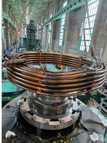
Removing pump unit cooling coil for repair
