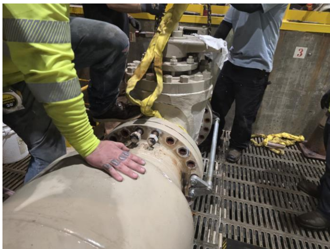
Staff dismantling pipe section (left) and hoisting pipe section out of Oak Street PCS (right)
