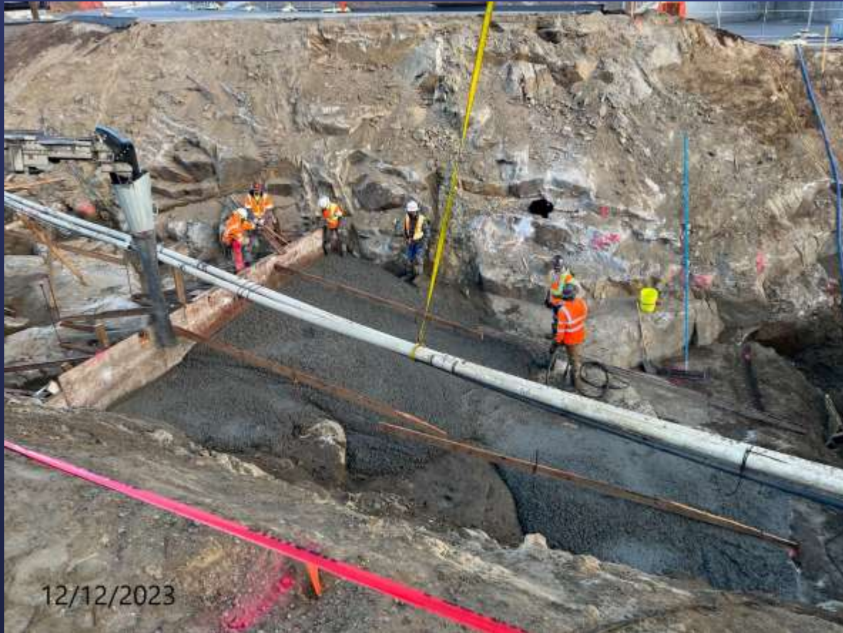
Pouring of Mass Concrete at 96" Pipe Tie-in
