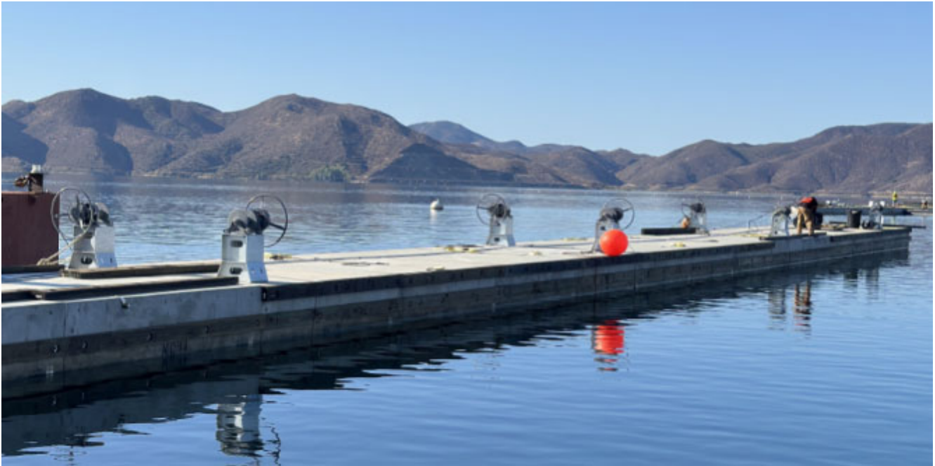
Diamond Valley Lake (DVL) Wave Attenuator Replacement — Installation of Winches on New Floating Wave Attenuator
