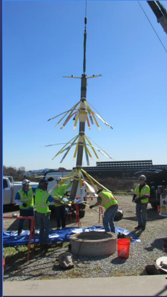
Prior Sepulveda Feeder Inspection
