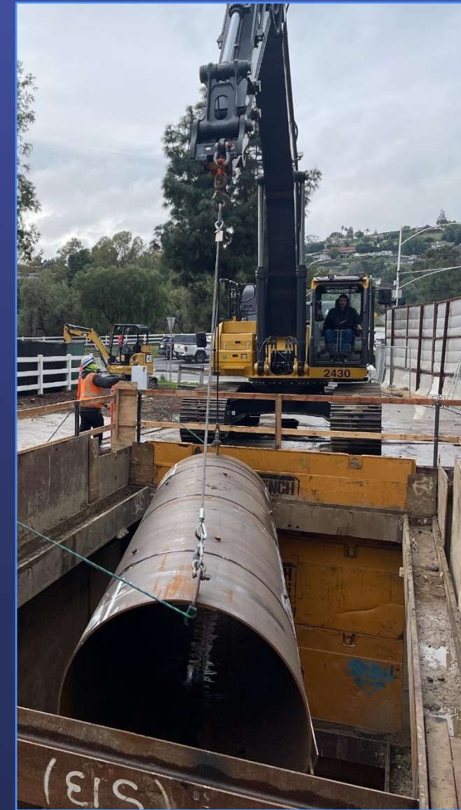
Second Lower Feeder Relining
