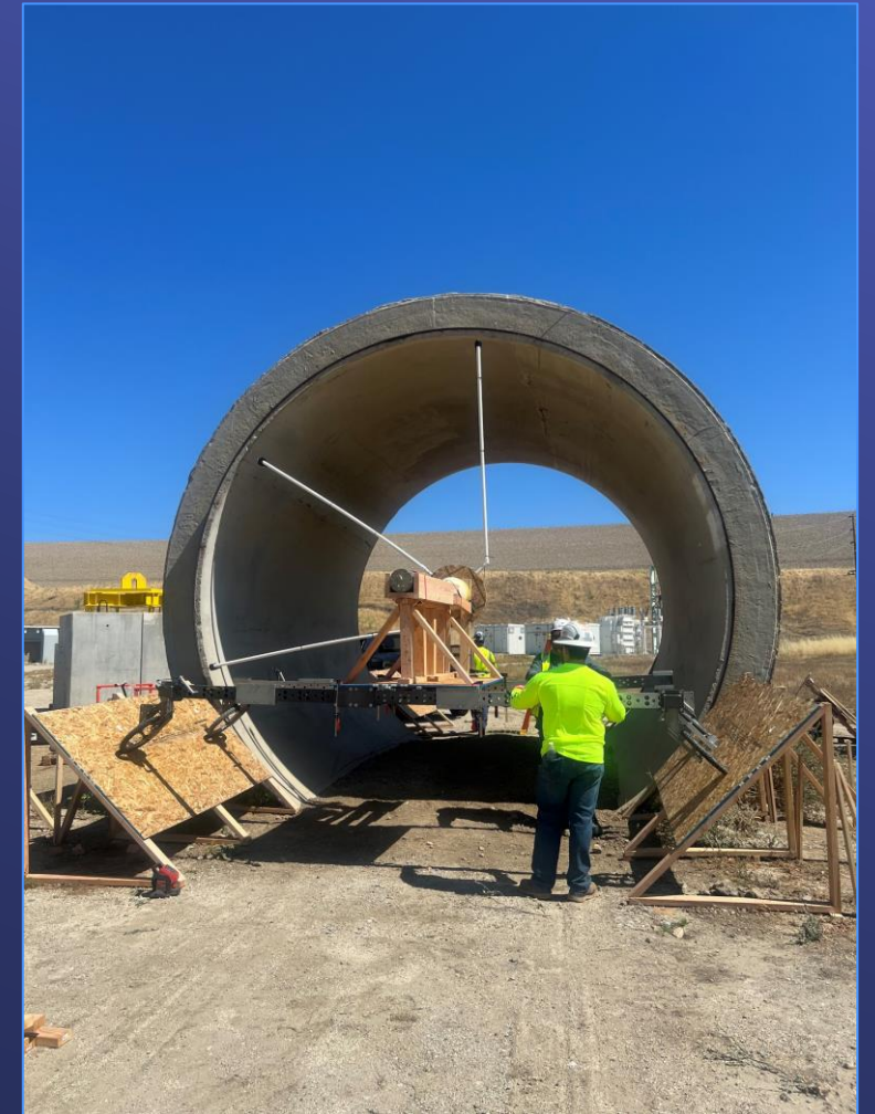
Calibration of PipeDiver tool for 201-inch diameter at Foothill PCS
