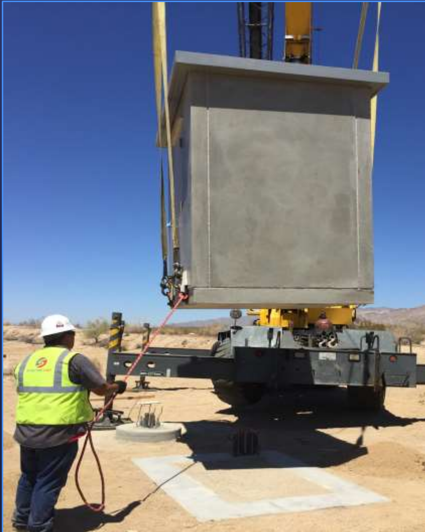
Typical pre-cast concrete building
