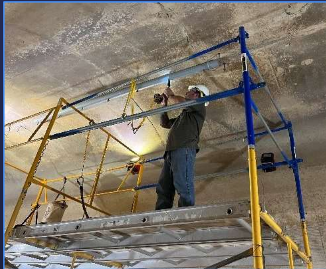
Typical transducer installation in aqueduct
