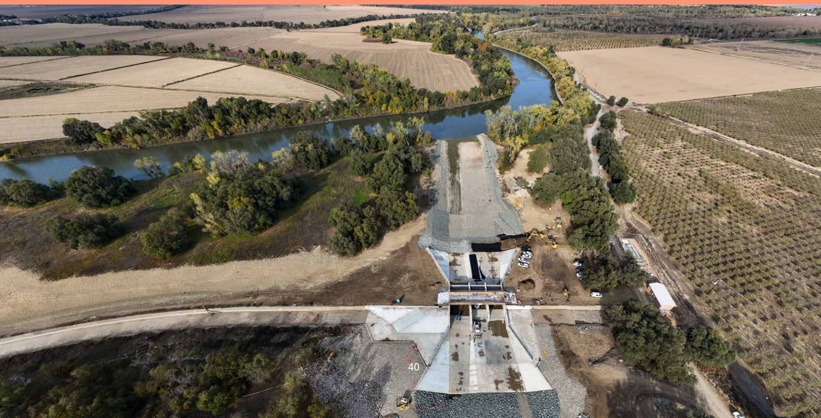
Drone view of Yolo Bypass Salmonid Habitat Restoration and Fish Passage (Big Notch) Project, courtesy CA Department of Water Resources.
