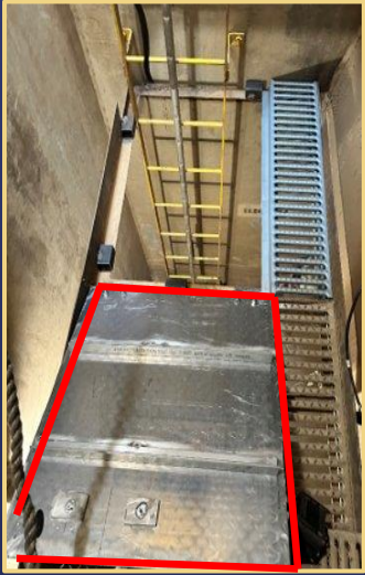
Yorba Linda Feeder Hinged Hatch Opening
