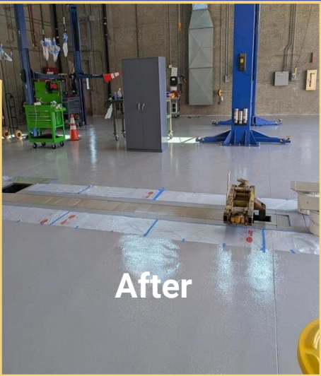
Anti-Slip Coating and Stencils
