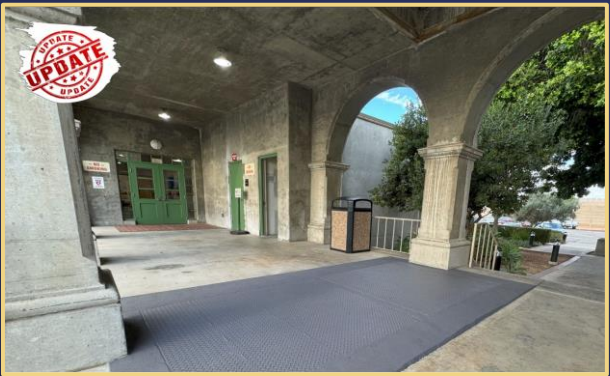
LV Breezeway Recoated and Fixed Trip Hazard
