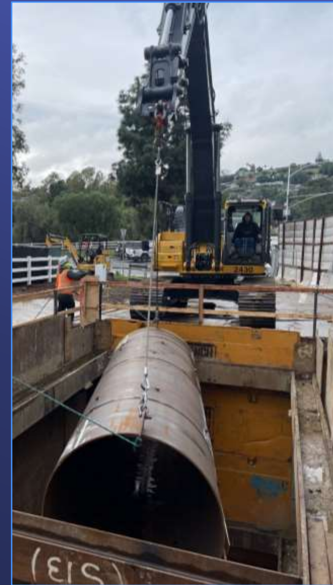
Second Lower Feeder Relining
