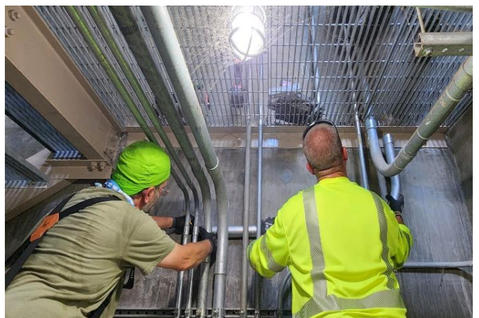
Routing conduit inside the structure
