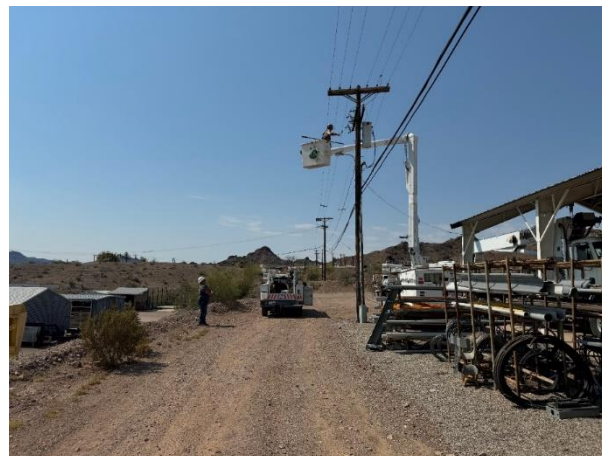
Staff replacing a 2300/480V transformer at the Gene pumping plant
