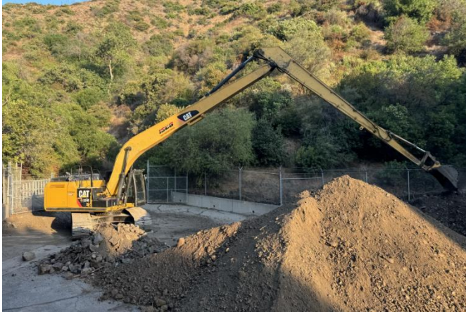
Long-reach excavator removing debris from catch basin
