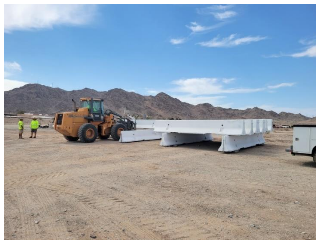
K-Rails to be used as 230kV tower protection
