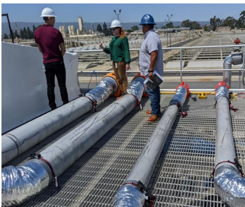
Installation of bioreactor materials in preparation for acetone spiking test at the NIC
