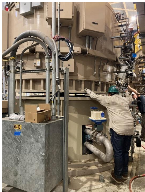
Staff removing motor for repairs at the Wadsworth pumping plant
