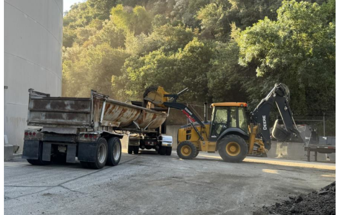
Backhoe loading truck with debris
