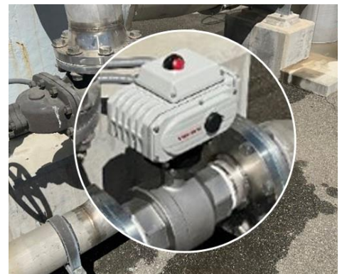
Open loop strainer valve, spool, and actuator (after replacement)
