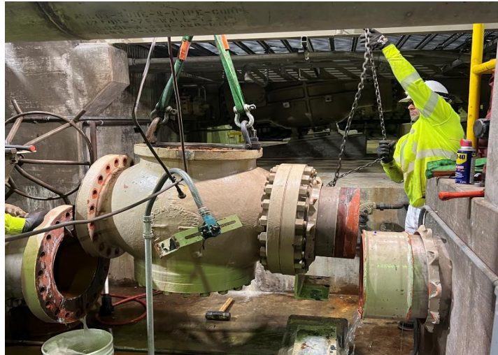
Staff repairing hydraulic globe valves at the Ramona PCS
