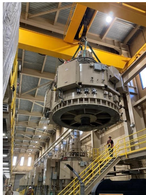
Staff removing motor for repairs at the Wadsworth pumping plant
