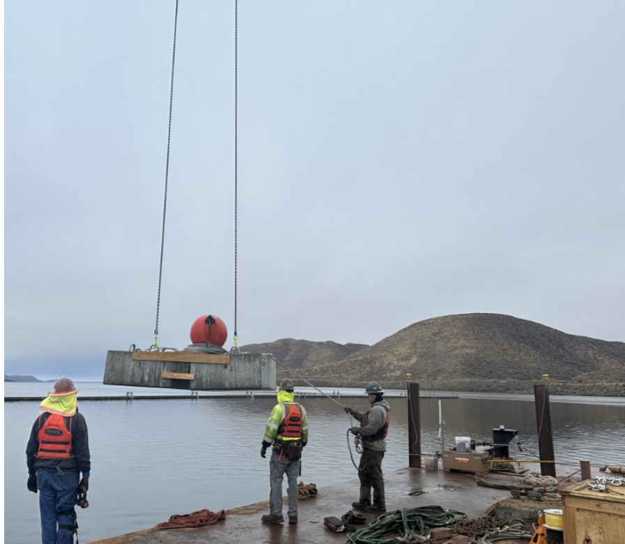
Diamond Valley Lake Wave Attenuator Replacement – Installation of Concrete Anchor Blocks
