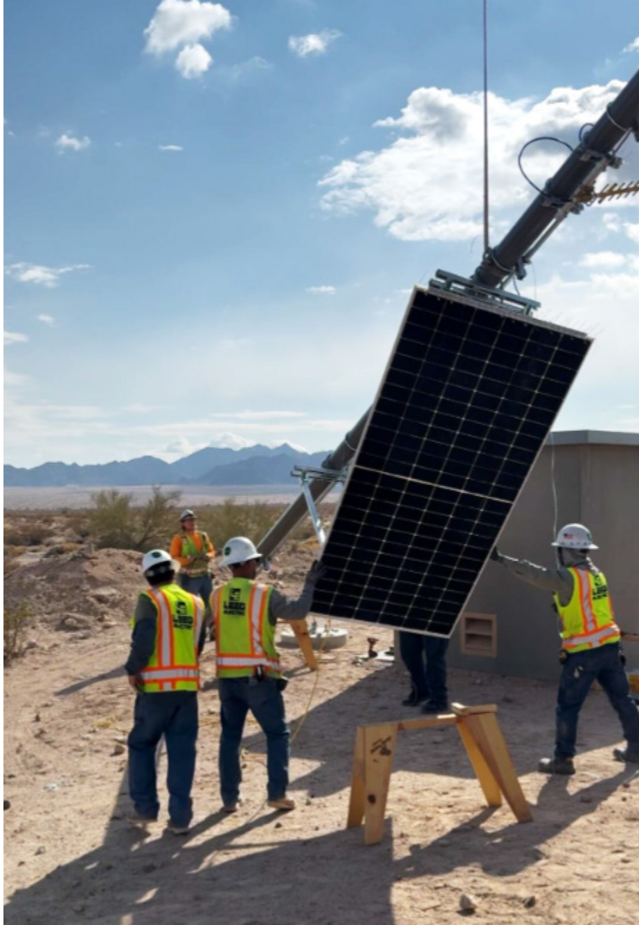
CRA Flow Level Monitoring Stations – Installation of Solar/ Antenna Pole
