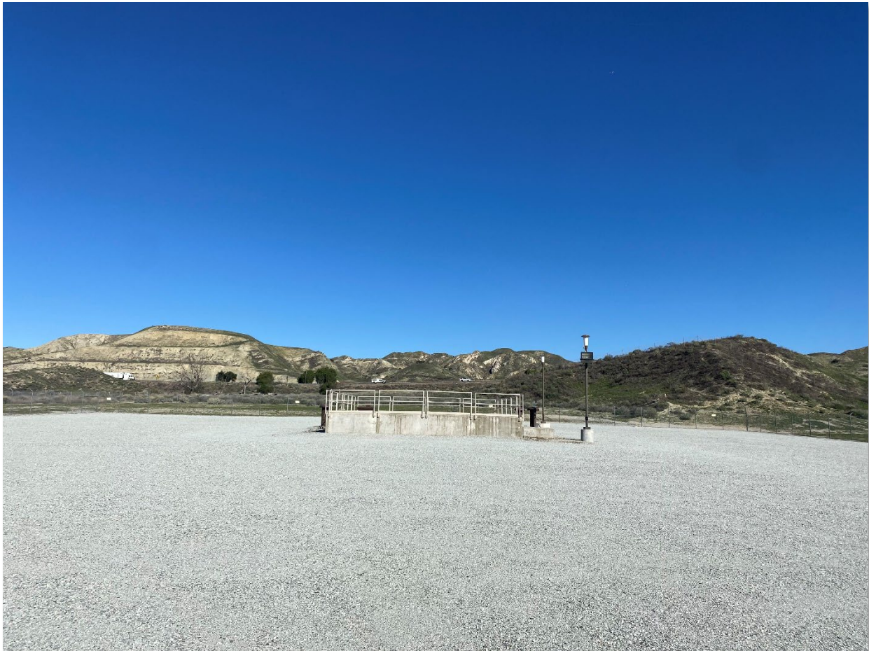
Badlands Tunnel south portal vault location on Inland Feeder
