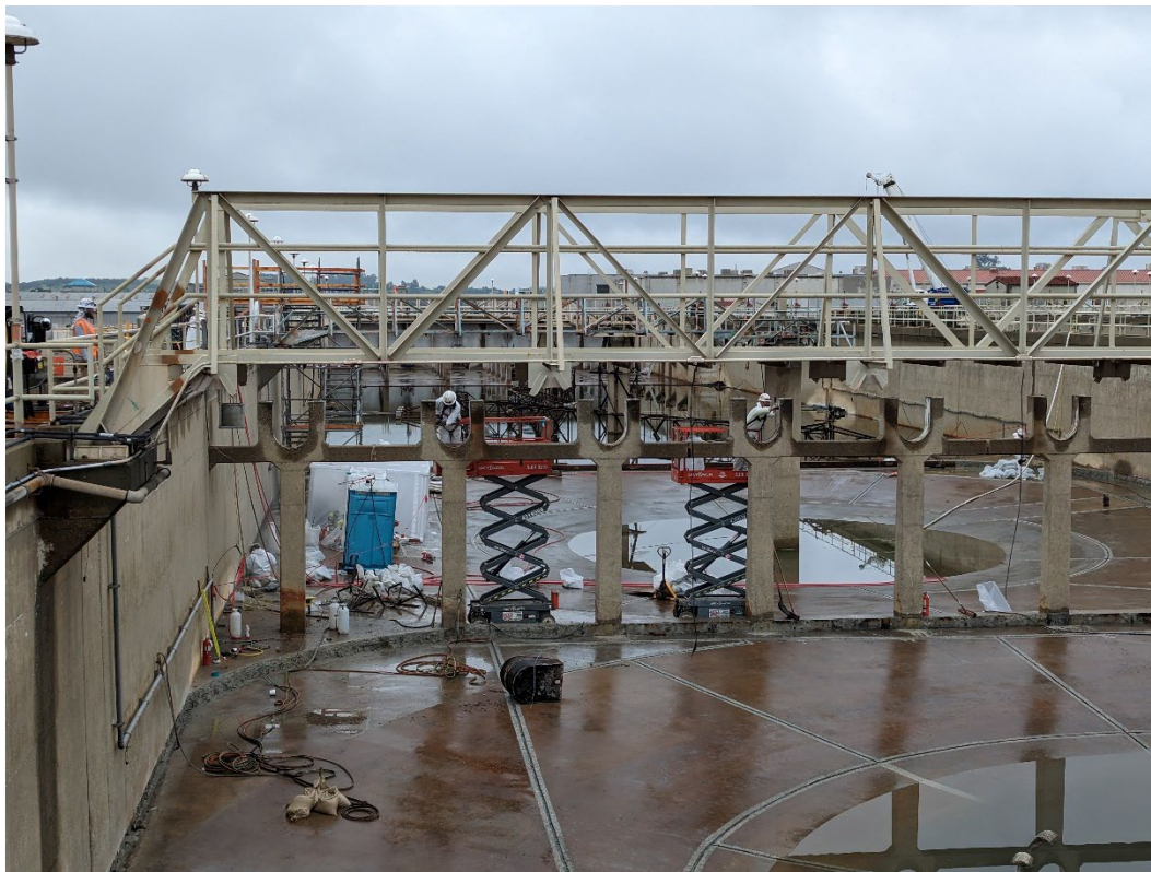
Weymouth Basin No. 8 launder trough demolition during the first quarter-plant shutdown
