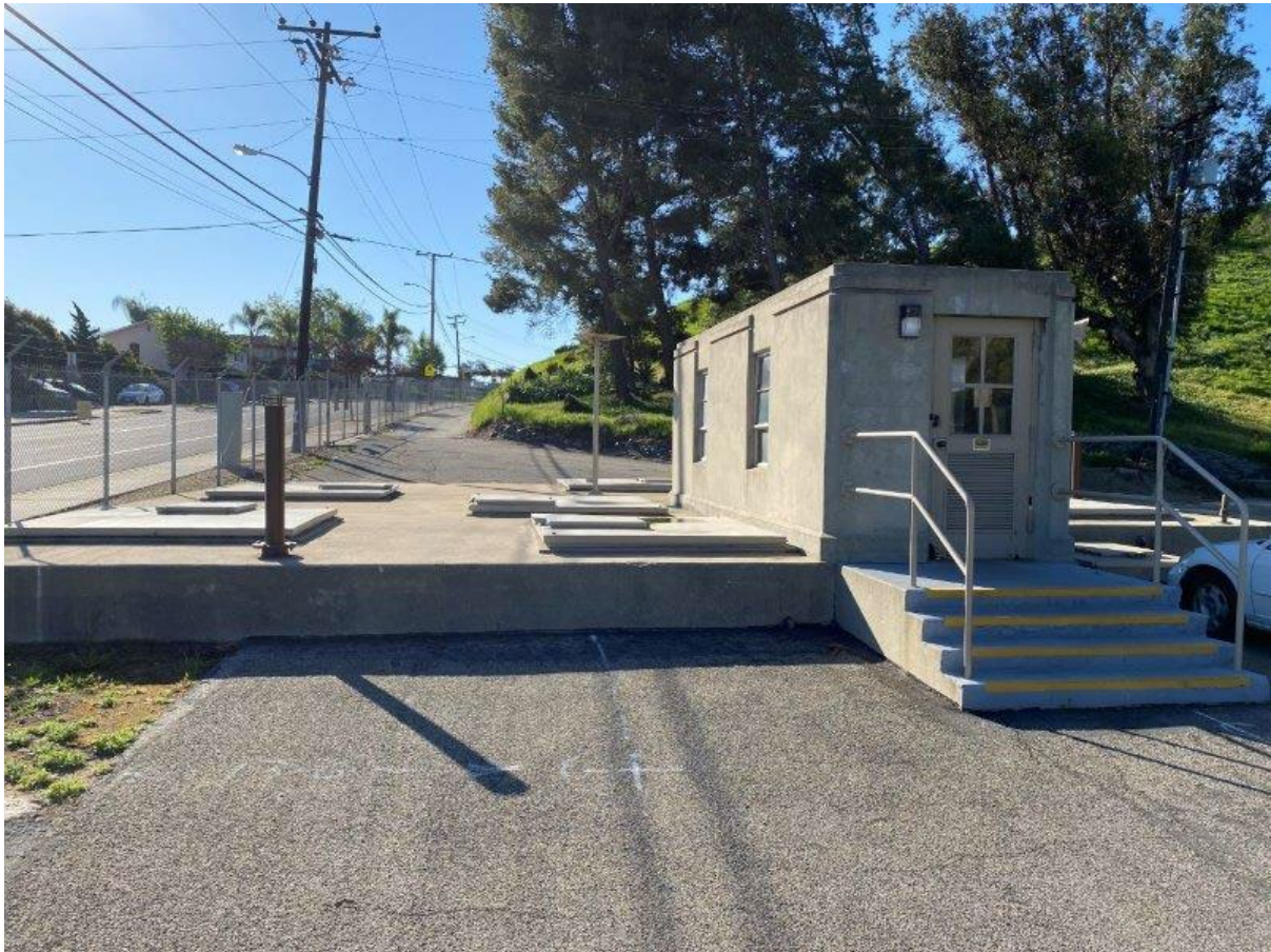
Exterior view of the Garvey Reservoir junction structure
