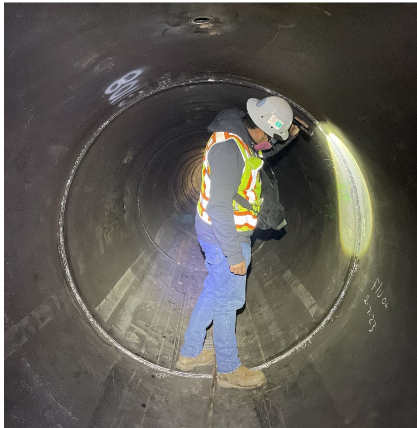
Inspection of new steel liner circumferential welds
