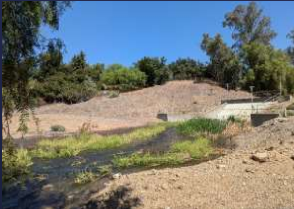
Spillway Flow Test
