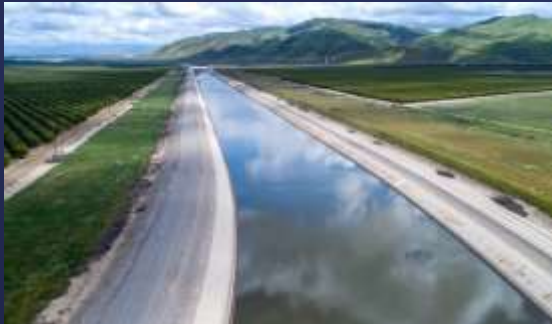
California Aqueduct in Central California
