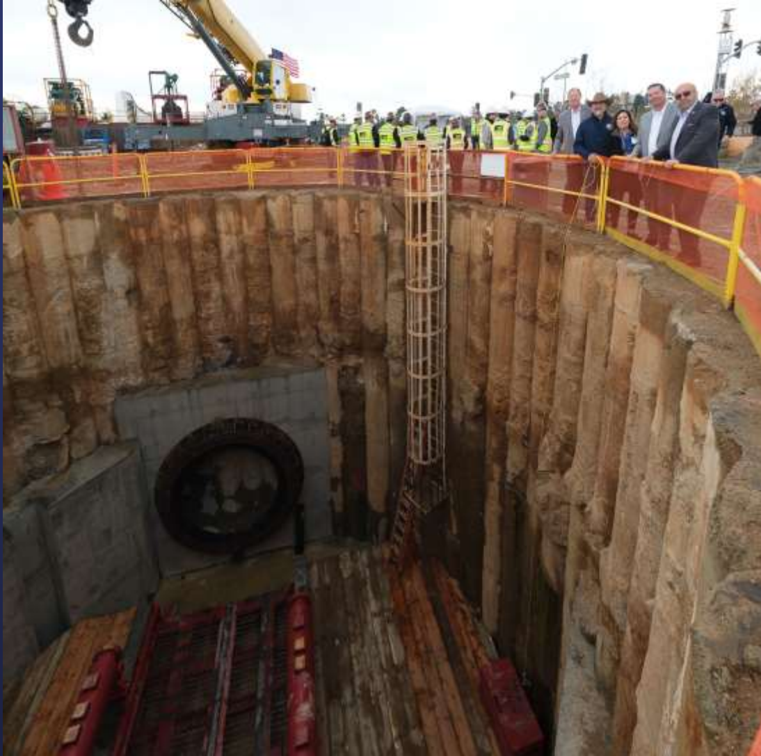
Tunnel Launch Shaft
