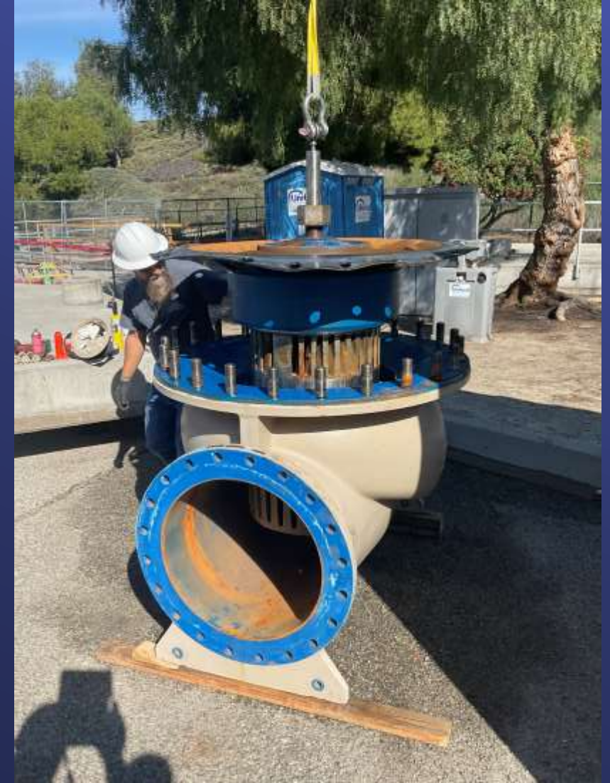
Inspection of 24-inch Cla Valve
