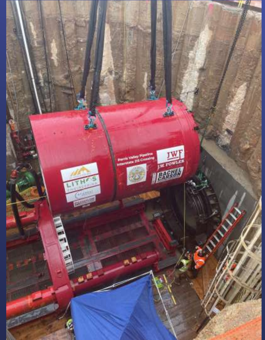
TBM Lowered into Launch Shaft
