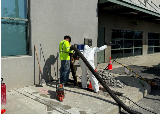
Staff excavating a gas line using Hydro-Excavation to prevent damage to utilities at the Weymouth plant
