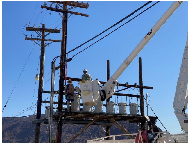
Staff performing repairs to an overhead electrical bank at Gene Camp
