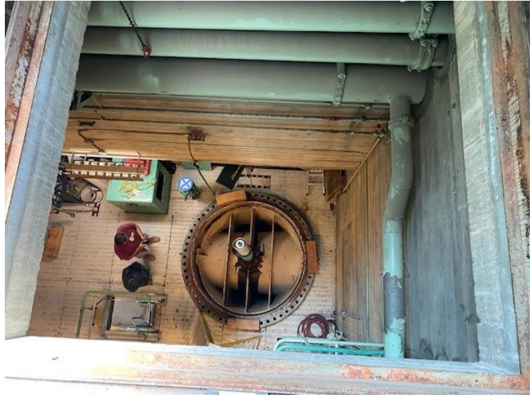
Discharge Valve repair at Gene pumping plant
