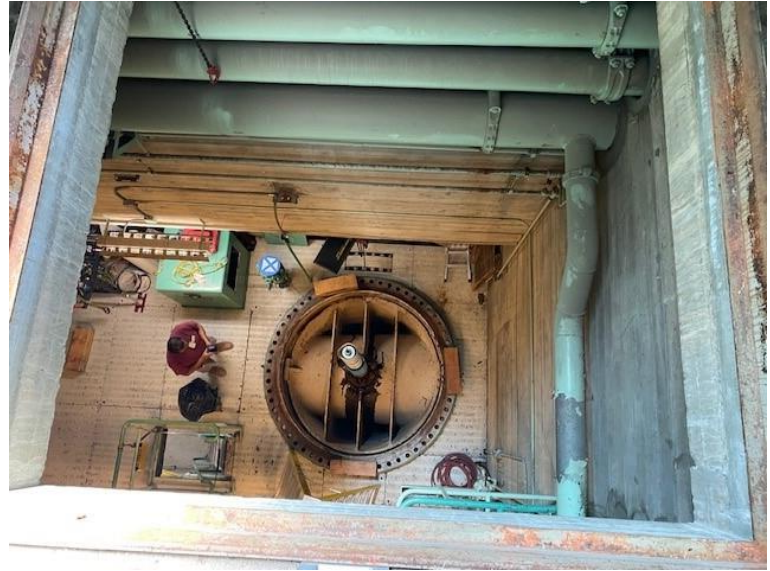
Discharge Valve repair at Gene pumping plant
