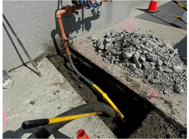
Staff excavating a gas line using Hydro-Excavation to prevent damage to utilities at the Weymouth plant
