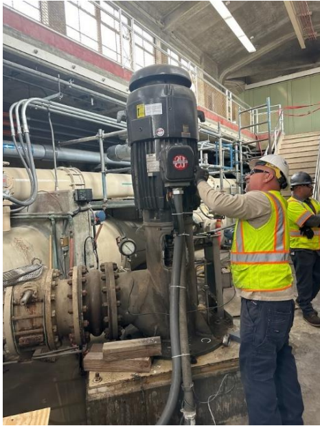
Terminating cables and programming the new ASDs to control pumps at the Weymouth plant
