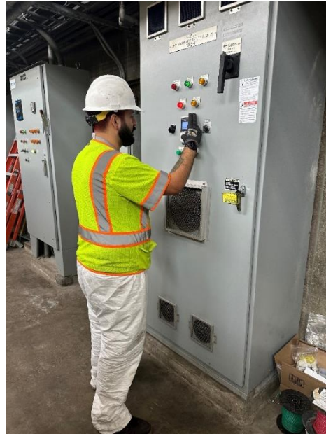
Terminating cables and programming the new ASDs to control pumps at the Weymouth plant
