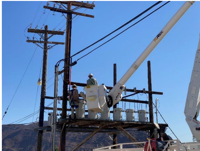
Staff performing repairs to an overhead electrical bank at Gene Camp
