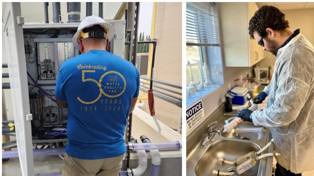
Electrical panel maintenance (left) and preparing ultrafilters for microbial sampling of the MBRs (right) at the NIC demonstration facility
