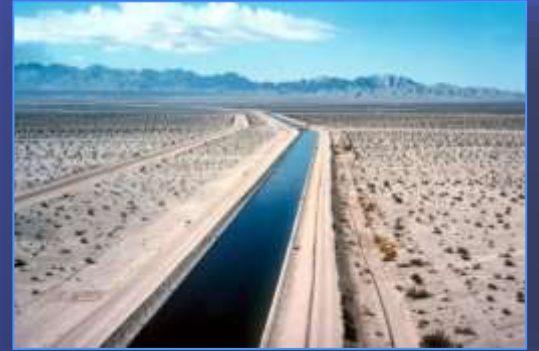
Colorado River Aqueduct
