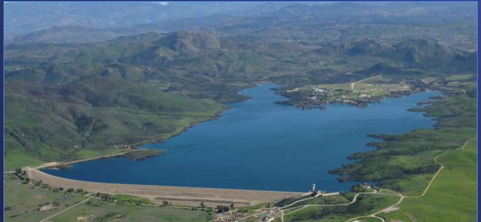
Lake Skinner (outlet tower lower right in photo)
