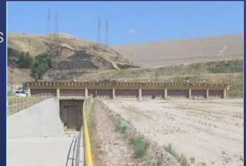
Foothill Control Building
